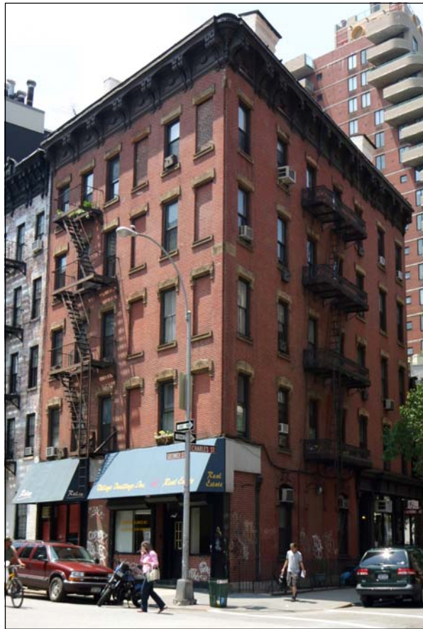
716-718 Greenwich Street aka 128 Charles Street
