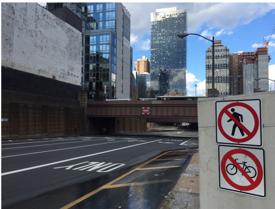
Figure 18: View of West 37th St bridge over Dyer Ave from West 38th St, photo: Brian Weber
