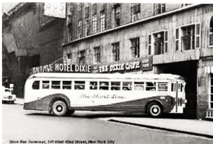
Figure 9: Dixie Bus Terminal, 241 West 42 nd St, 1930, image from scoutingny.com
