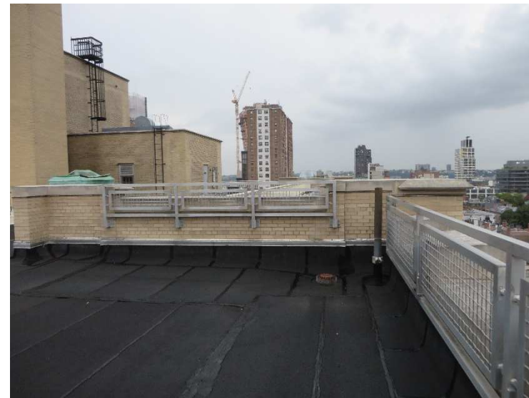
Membrane coating and patching in many locations
