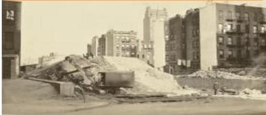
Demolition on West 35 th Street and 9 th Avenue for the construction of Dyer Avenue
