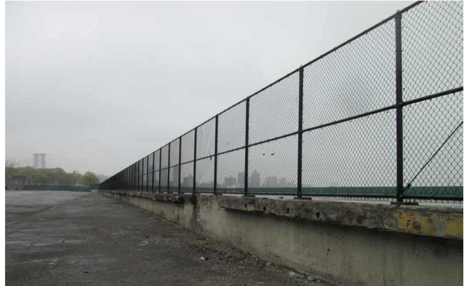
4 View of existing 8' height chain link fence at deck perimeter.
