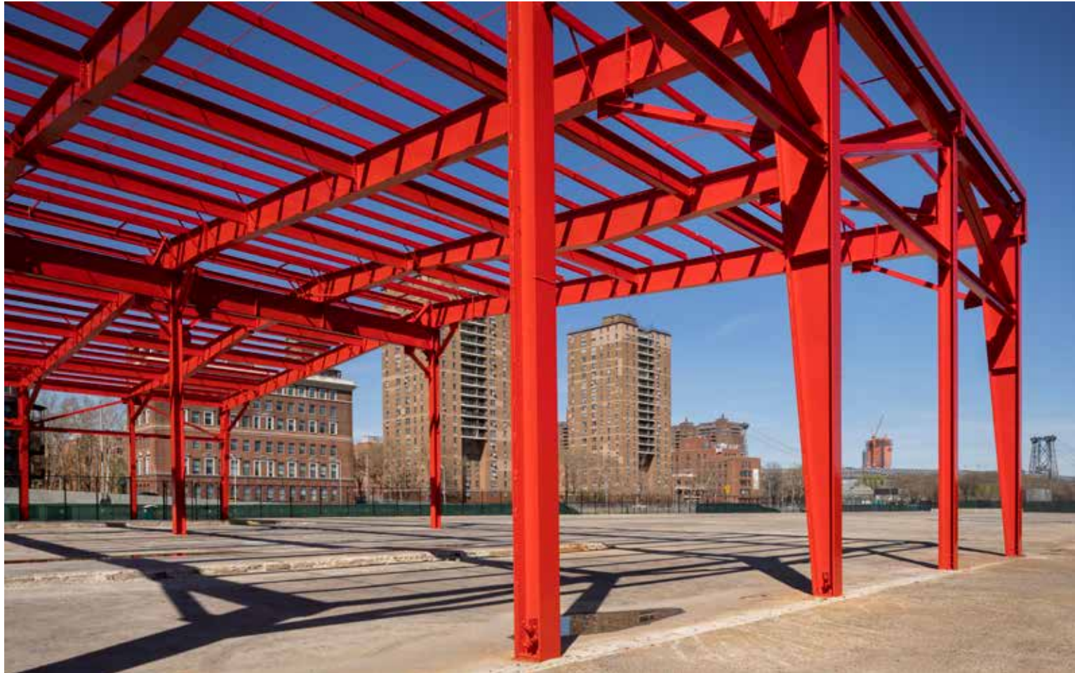
3 View northeast with raised concrete slab visible beneath the structure.
