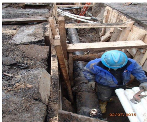
Cooper Sq. West: Newly installed 12" Water Main Pipe
