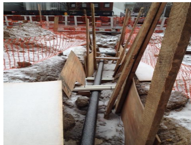
Village Plaza: Partial Installation of fire hydrant branch
