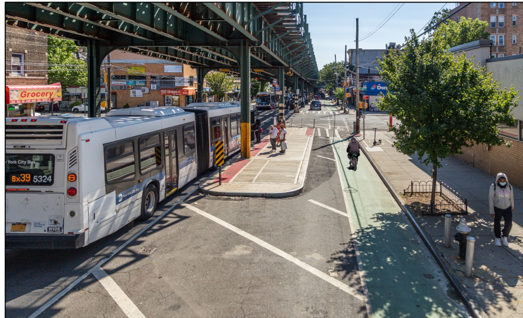
Protected Bike Lane and bus boarding island installed in 2022 on White Plains Rd
