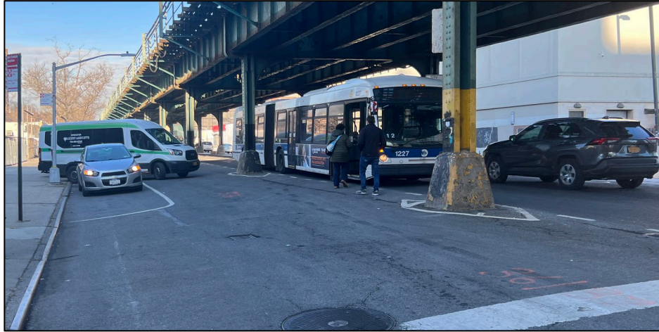
Existing Conditions at White Plains Rd and Waring Ave
