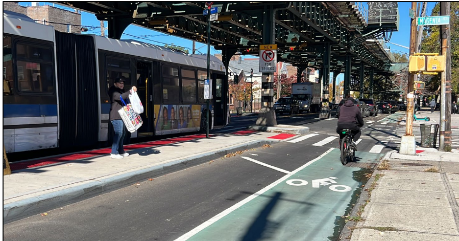
Completed Bus Island at White Plains Rd and Magenta St
