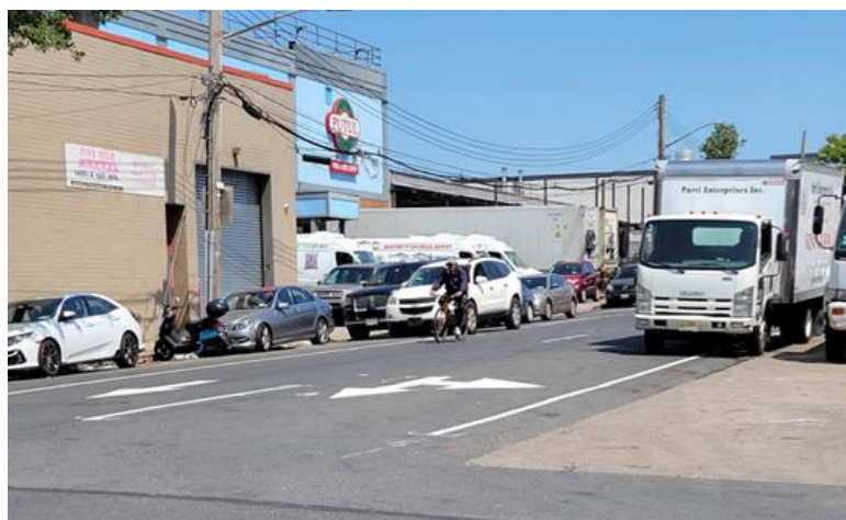
Figure 29: Pavement markings refurbishment on an industrial street in Maspeth IBZ
