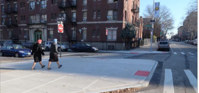
Proposed condition (concrete curb extension) for multiple intersections along 3 rd Ave (Photo: Willoughby Ave)
