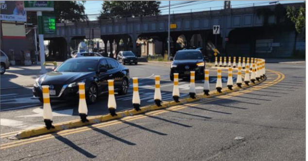
Proposed condition (hardened centerline) for multiple intersections along 3 rd Ave (Photo: Hempstead Ave)
