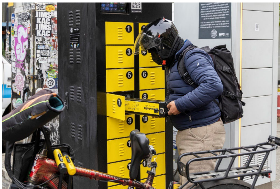
Electric Bikes Charging Stations at Cooper Square, Manhattan
