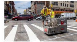
200M linear ft of markings
