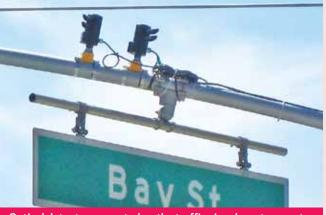
Optical detectors mounted on the traffic signal mast arms at 14 intersections along the study area receive requests form approaching buses.
