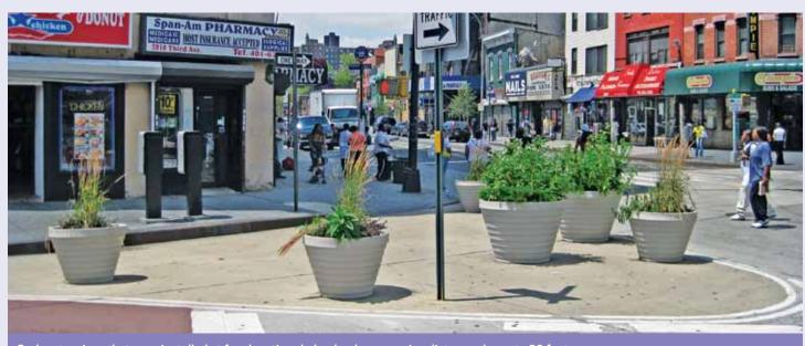
Curb extensions that were installed at four locations helped reduce crossing distances by up to 20 feet.
