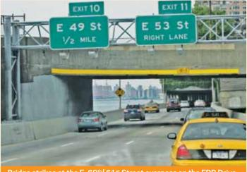
Bridge strikes at the E.  $60^{th}/61^{st}$  Street overpass on the FDR Drive are down 56% since the treatment was installed, the greatest reduction of any pilot location.
