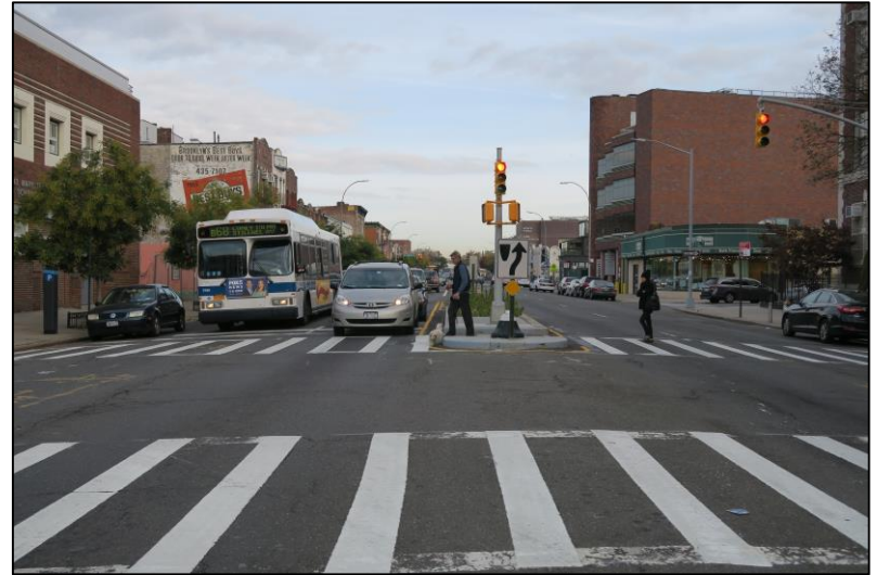
Pedestrian refuge island; Coney Island Ave and Ave N
