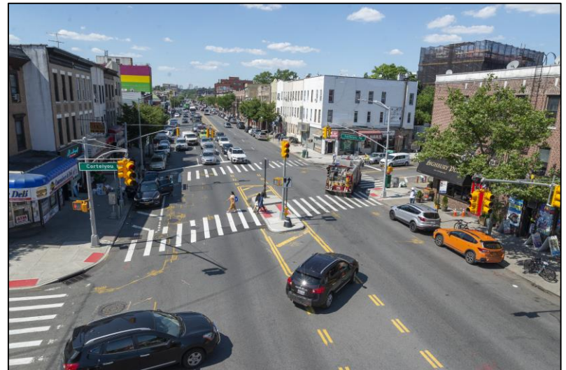
Pedestrian island and new crossing; Coney Island Ave and Cortelyou Rd
