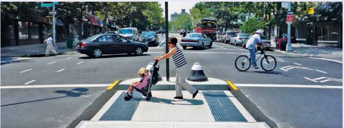
Refuge islands and a landscaped median improve the environment for this retail and pedestrian corridor.
