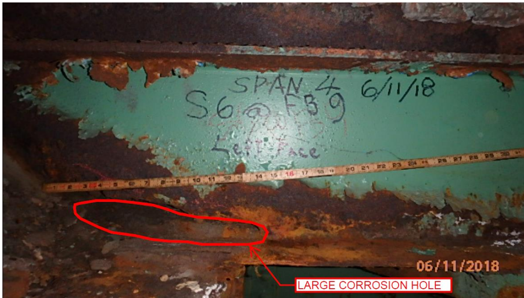
Figure 1: Stringer exhibiting large corrosion holes and severe section loss along interface to concrete counterweight. Source: 2018 NYSDOT Biennial Inspection Report
