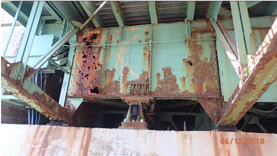
Figure 3: Span 4, west leaf, Floorbeam FB1 between Truss T3 and T4, exhibiting numerous corrosion holes and severe section loss. Source: 2018 NYSDOT Biennial Inspection Report
