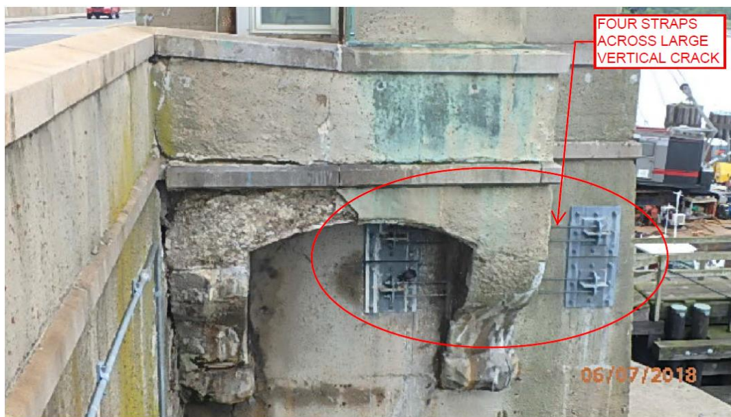
Figure 9: Spalled and cracked concrete in left parapet along the side of the Operator's house. Note the large vertical crack along the side of the Operator's house supported by four steel straps (tensioning members) anchored to the side of the Operator's house to prevent further expansion of the crack. Source: 2018 NYSDOT Biennial Inspection Report
