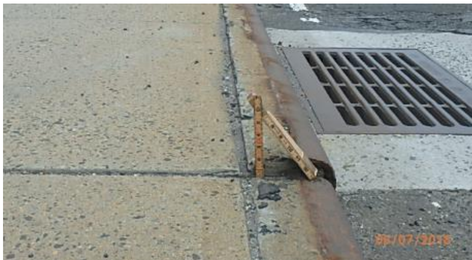
Figure 5: Differential elevation between the curbs at Span 3.
