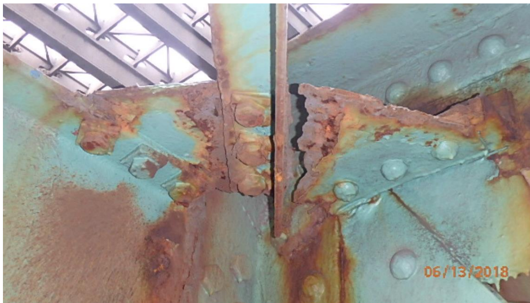
Figure 4: Right side of Truss T2, connecting to Floorbeam FB5, exhibits completely broken gusset plate along T2. Source: 2018 NYSDOT Biennial Inspection Report
