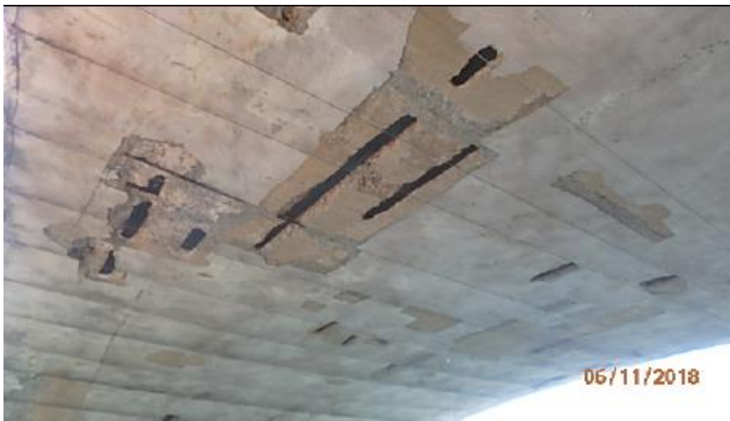
Figure 6: Span 5 underside exhibits spalled and hollow sounding concrete on arch intrados. Source: 2018 NYSDOT Biennial Inspection Report
