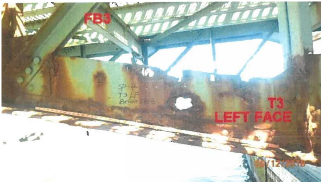
Figure 2: Corrosion holes and severe section loss on bottom chord vertical plate of Truss T3 Source: 2018 NYSDOT Yellow Flag NB185QW015
