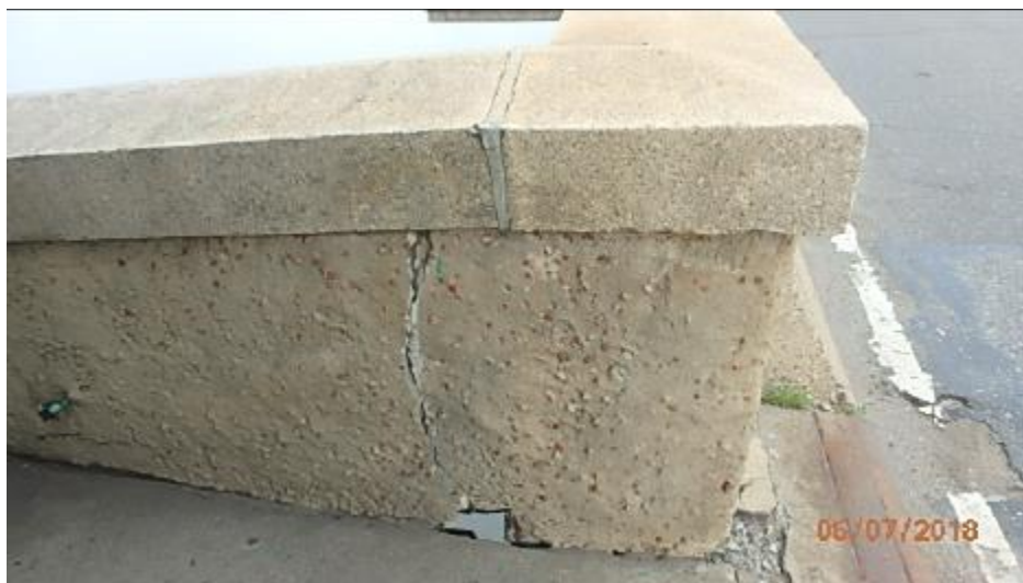
Figure 7: Parapet at Pier 4 along the side of the operator house exhibits a wide vertical crack with a hole at the bottom.
