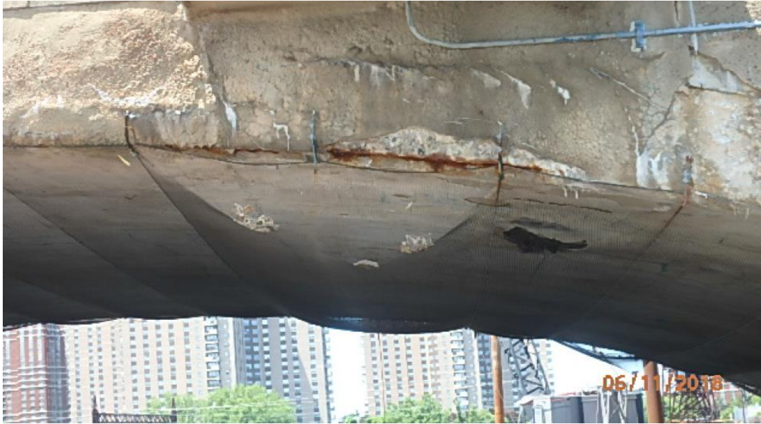
Figure 8: Typical deterioration at underside of arch spans. Note the small chunks of concrete that fell (at Span 3 near Pier 3) on nylon mesh netting covering entire arch intrados. Source: 2018 NYSDOT Biennial Inspection Report
