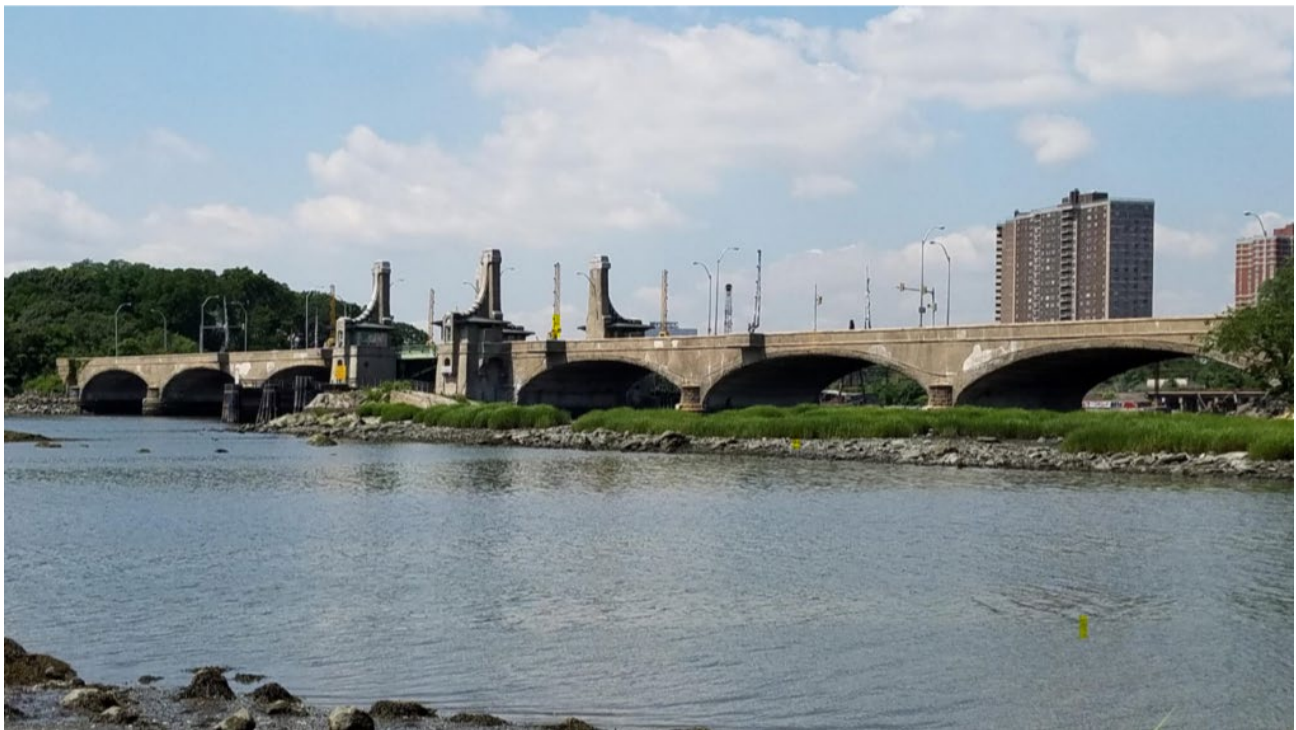
Figure 1. Shore Road Bridge (Source: NYCDOT)
