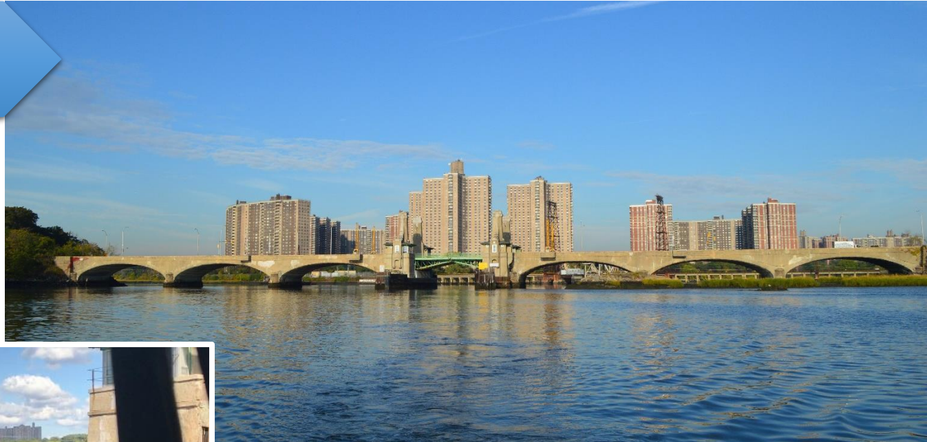
South Side of Bridge Looking North
