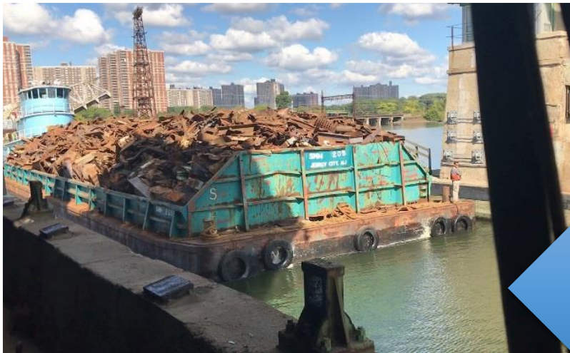
Barge In Narrow Bridge Channel
