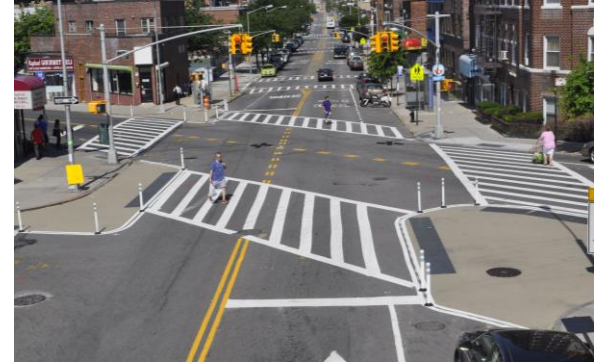
Proposed condition (painted curb extensions) for various intersections on Rochester Avenue (Photo: Greenpoint Ave and 48 th Ave, QN)
