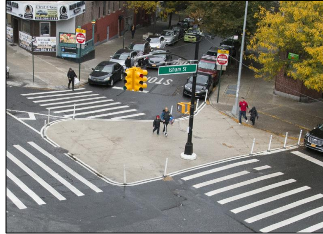
Painted Pedestrian Space with Flexible Delineators
