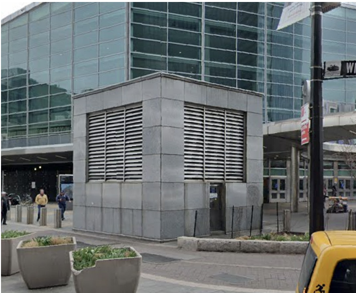
Figure 4.41 One of four ventilation structures for the Battery Park Underpass
