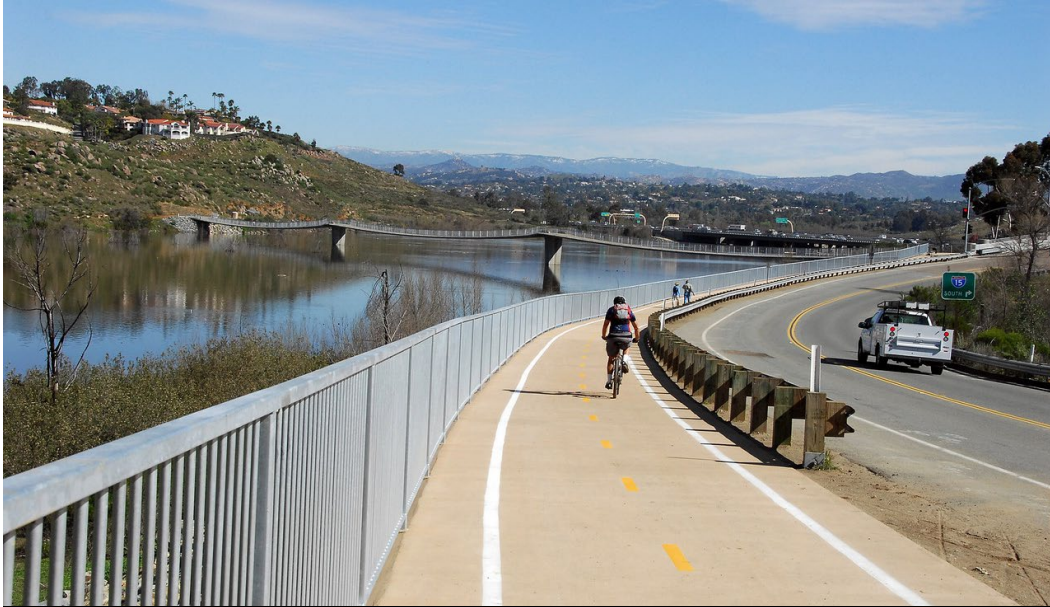
Proposed: West Bernardo Dr. Bike Path (cantilever structure) San Diego, CA
