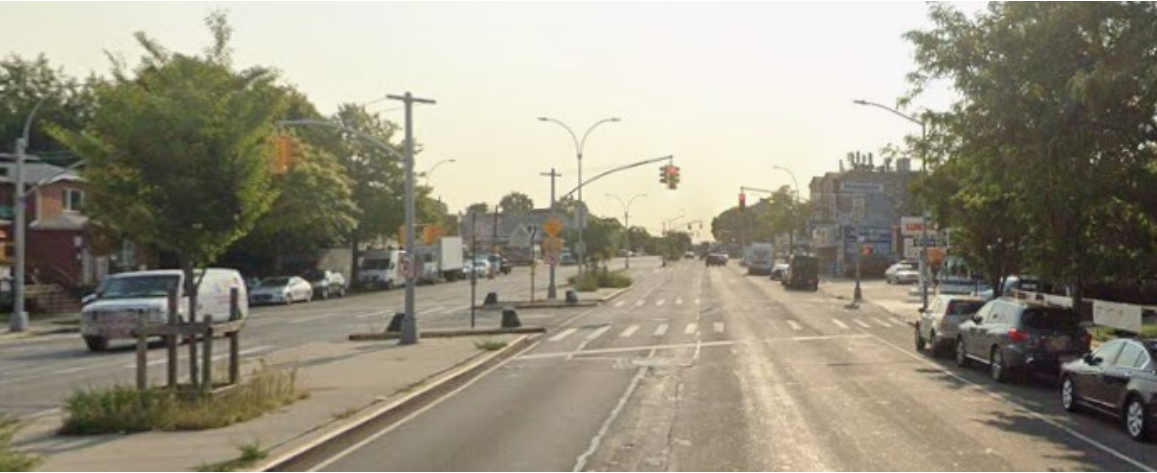
Existing: Astoria Blvd, looking east (90')
