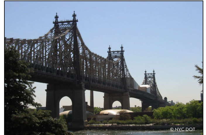
Ed Koch Queensboro Bridge
