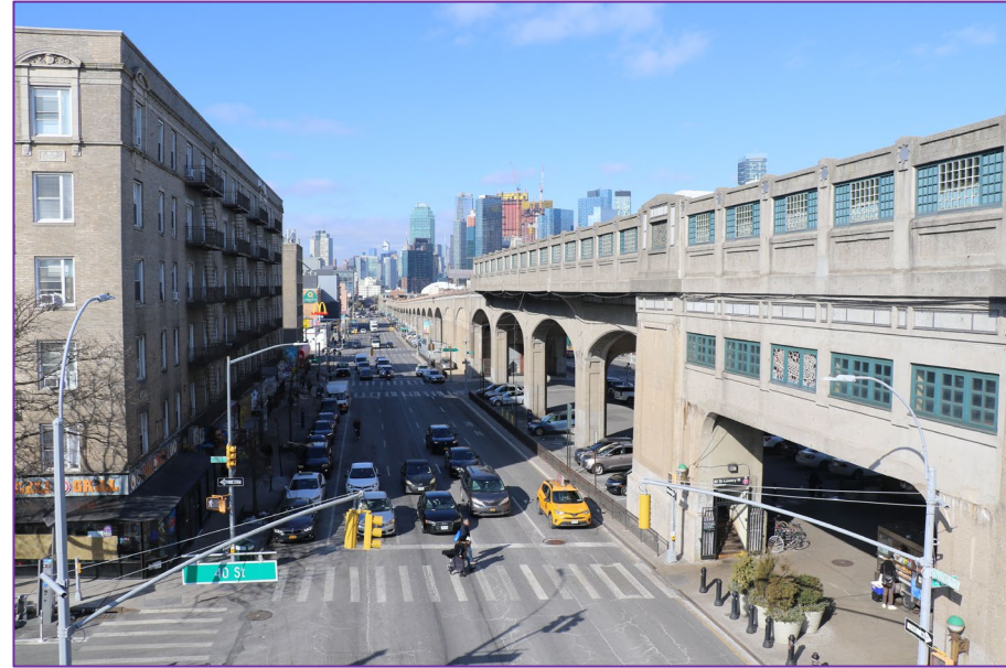
Queens Blvd at 44 th St
