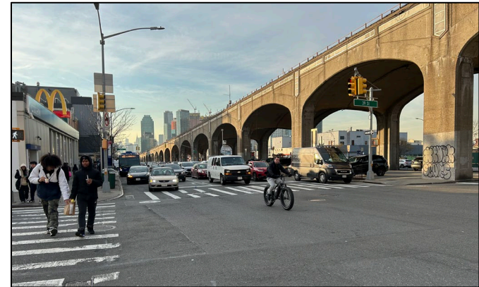
A taxi turns left onto Queens Blvd at 39 th St in front of a pedestrian; above. Pedestrians, a cyclist, and drivers on Queens Blvd, below
