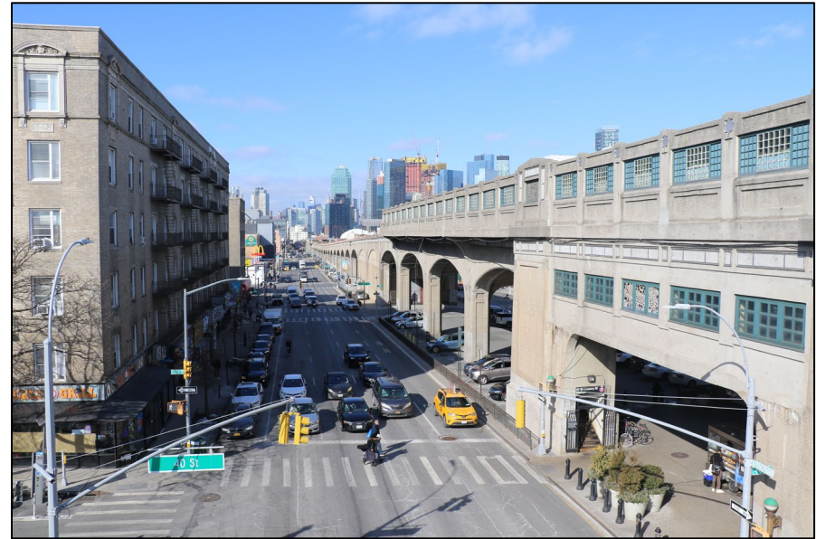
Queens Blvd at 40 th St, looking west
