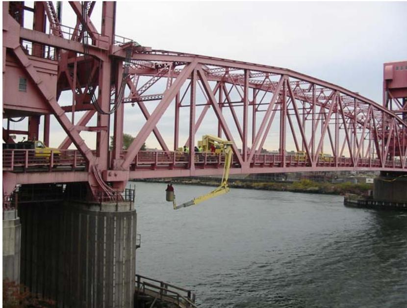
Bridge Inspectors in Sloop Under the Roosevelt Island Bridge (Credit: Bojidar Yanev)
