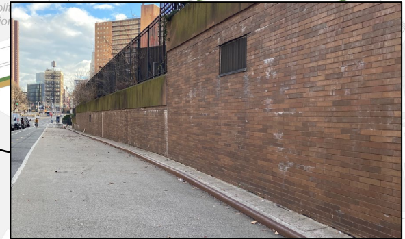
Lack of Wayfinding Signs on Park Row
