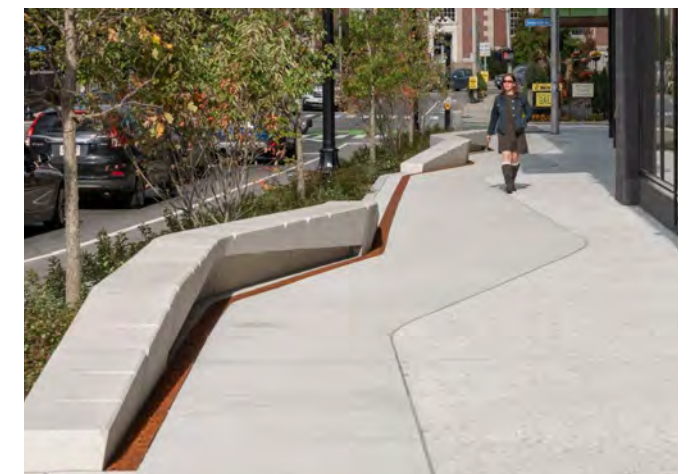
Cast-in-Place Concrete Union Square Station Plaza, Somerville MA
