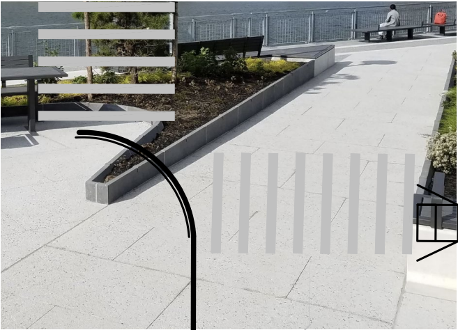
Large format pavers Greenpoint Landing
