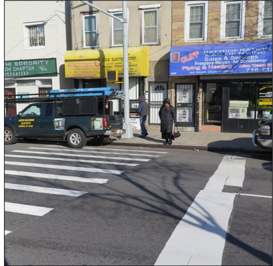
Missing pedestrian ramps and median cut-throughs
