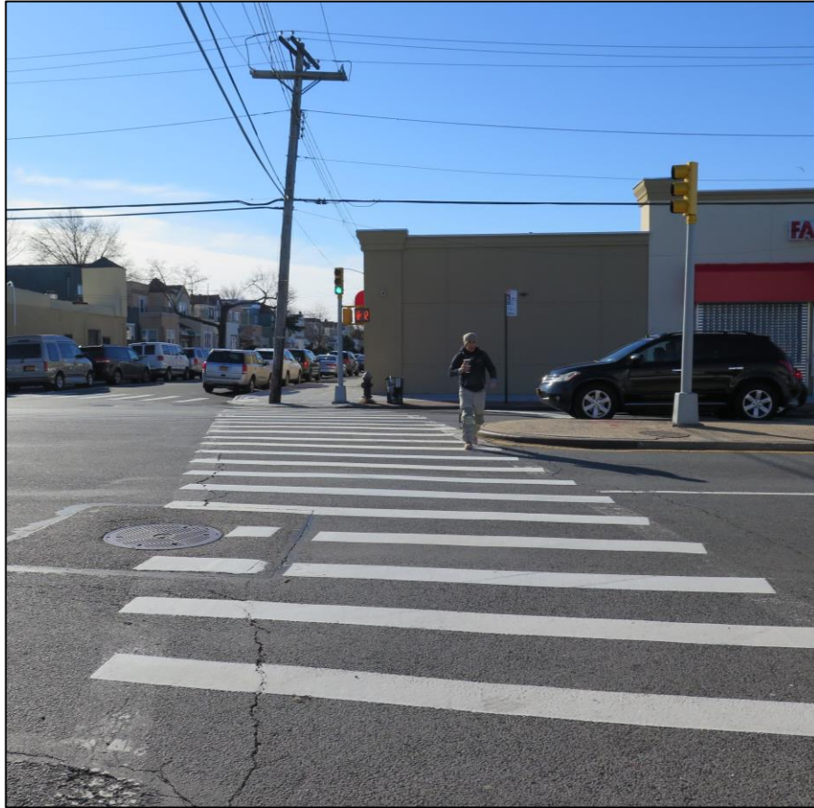
Long crossing distances and lack of pedestrian refuge space
