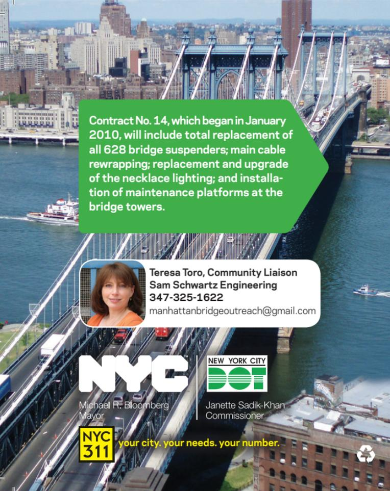
Contract No. 14, which began in January 2010, will include total replacement of all 628 bridge suspenders; main cable rewinding; replacement and upgrade of the necklace lighting; and installation of maintenance platforms at the bridge towers.
