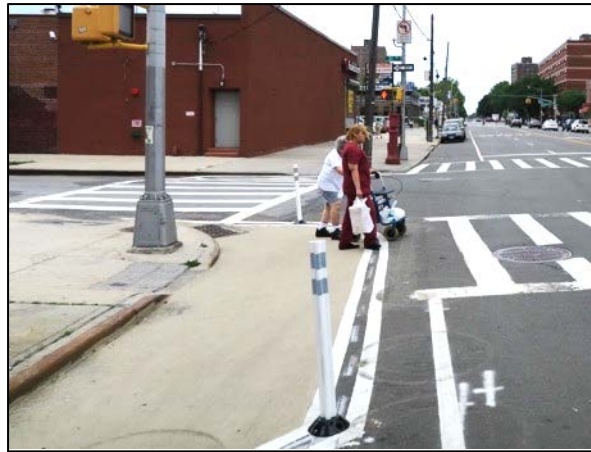
Painted Curb Extension with Flexible Delineators
