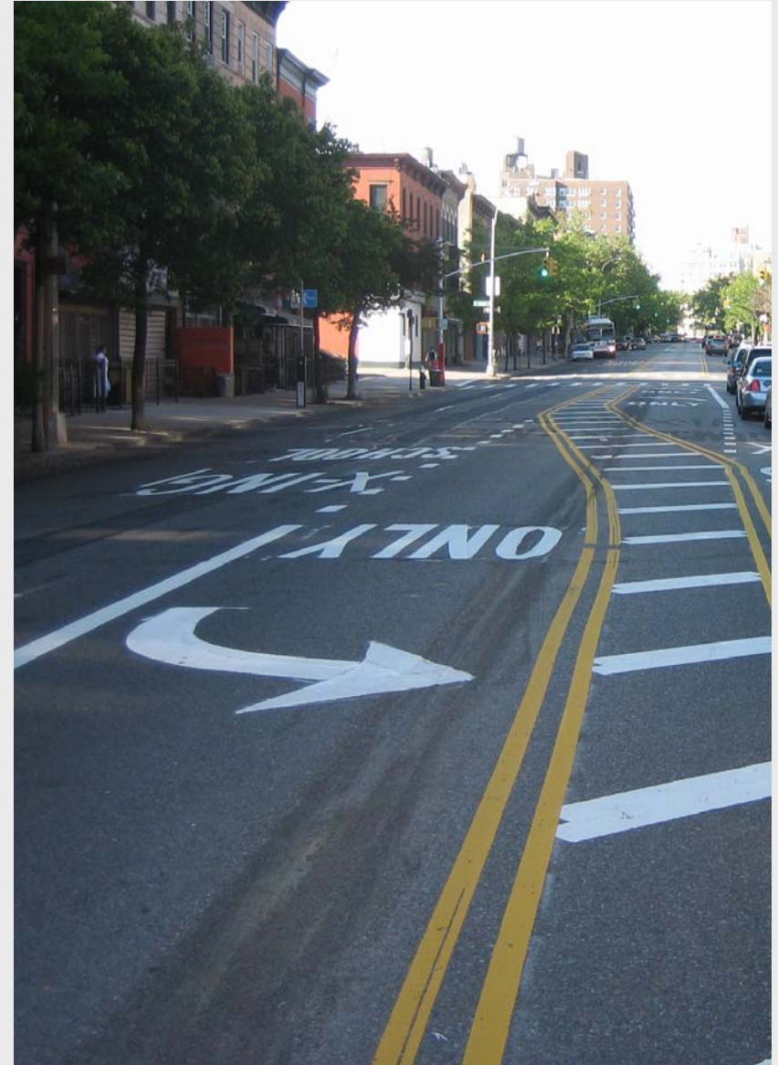
Left Turn Bays: Vanderbilt Avenue, Brooklyn
