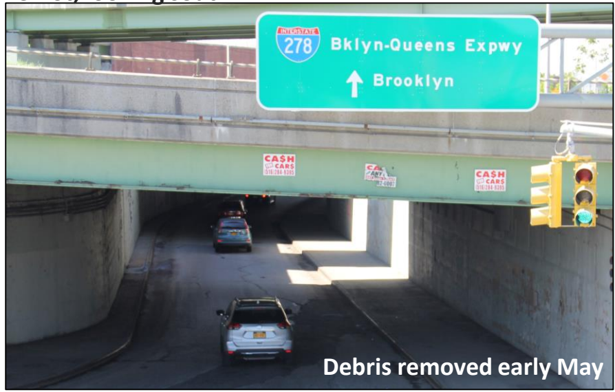
43 rd St, looking south
