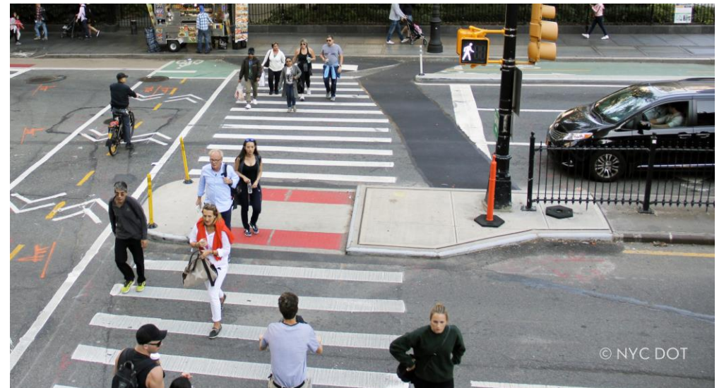
Proposed Condition (median tip extension) for multiple intersections along Kissena Blvd (Photo: Spruce St and Park Row, Manhattan)
