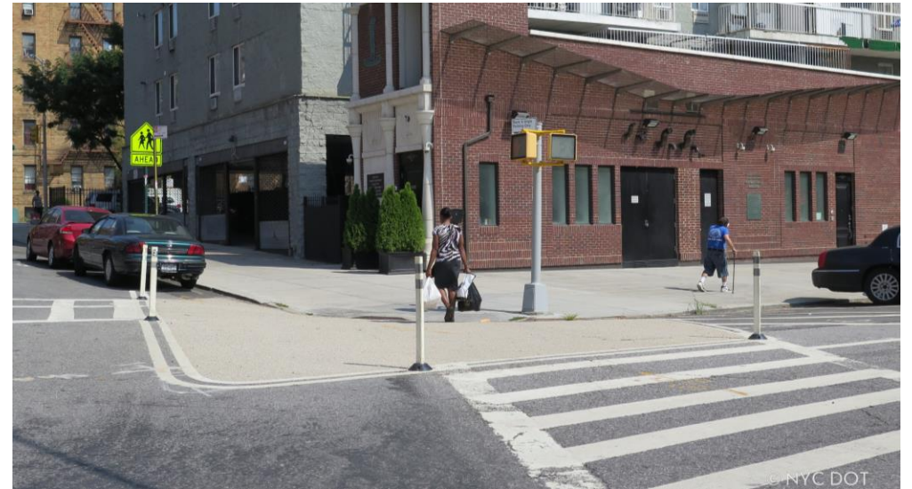
Proposed Condition (painted curb extension) for multiple intersections along Kissena Blvd (Photo: Troy Ave and Lefferts Ave, Brooklyn)
