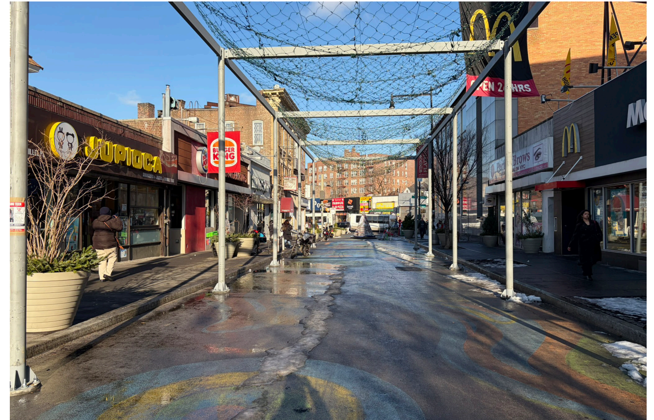
6 - A shade structure at the end of the street, approximately 24 feet wide by 80 feet long, accompanied by a mural graphic on the asphalt paving
