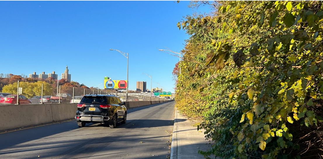
Existing: view of Sedgwick Ave, looking north
