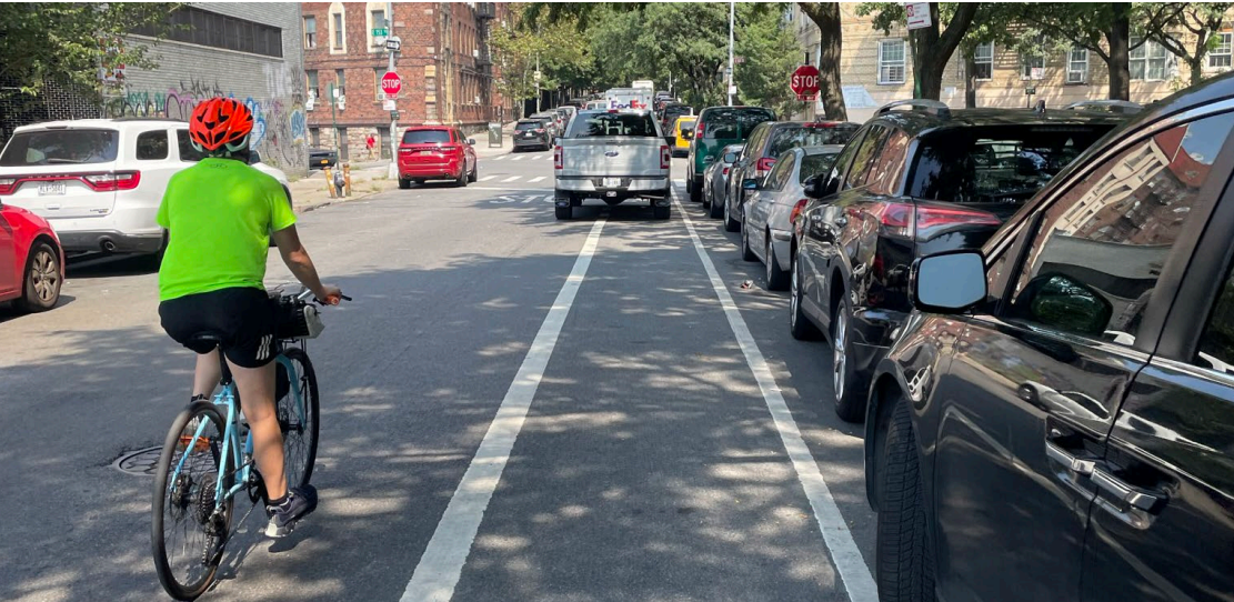
Existing: Gerard Ave at E 153 rd St, looking north – 34' wide
