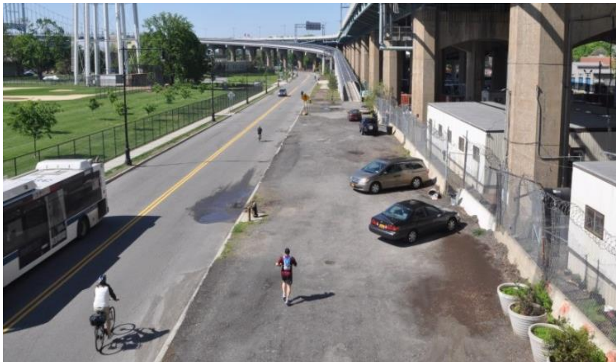
Existing: Hell Gate Cir, facing south
