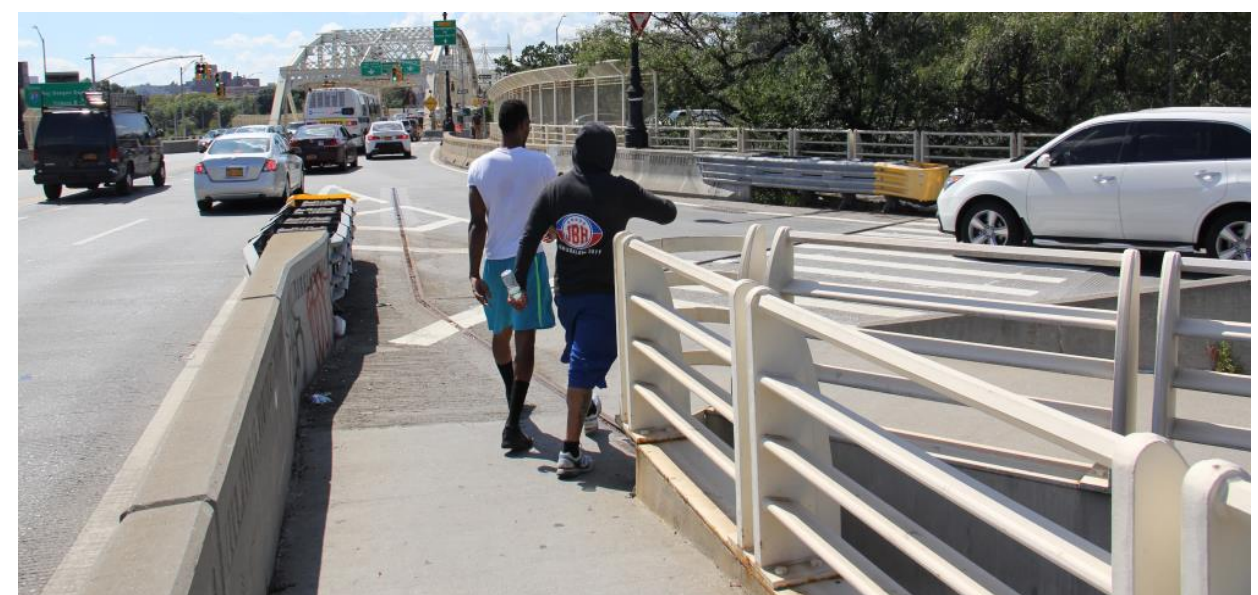
Existing: Macombs Dam Bridge, facing west
