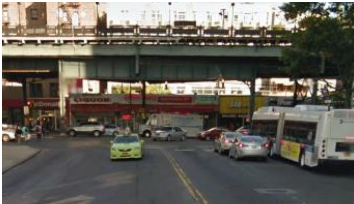
Existing: W 225 th St, Bronx facing west
