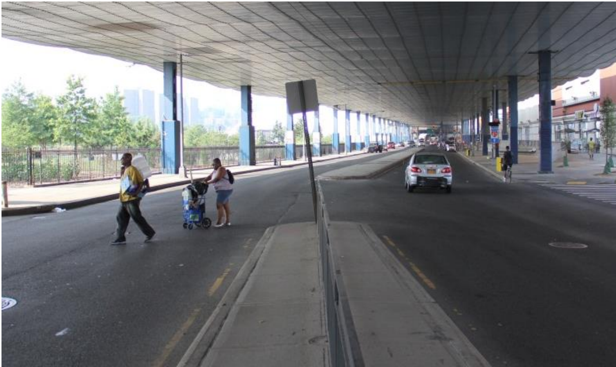
Existing: Gateway Center Blvd, facing northeast
