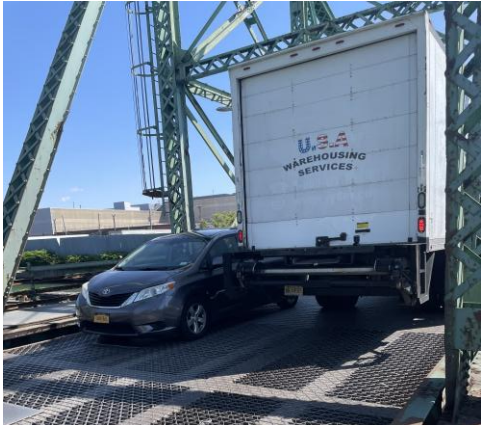
Typical Condition with Traffic on the Bridge
