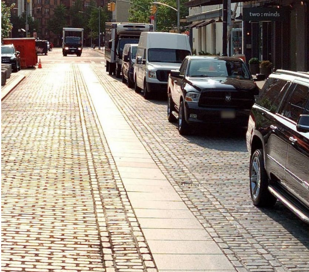
Completed granite bike lane on Gansevoort Street
