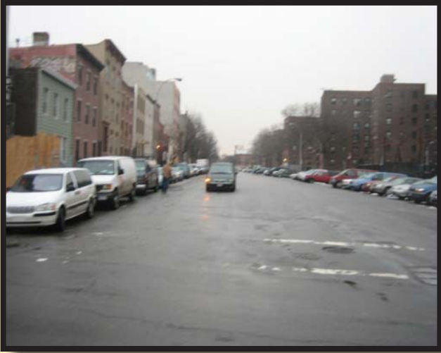
Conditions on Carlton Avenue prior to improvements.
