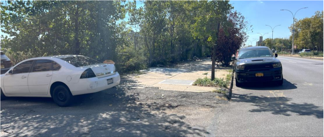
Missing pedestrian ramps
