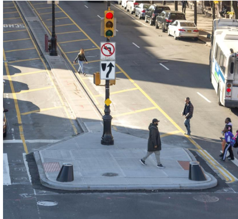
Proposed conditions (widened median with warning strips) for Fountain Ave (Photo: E 149th St and Grand Concourse, BX)
