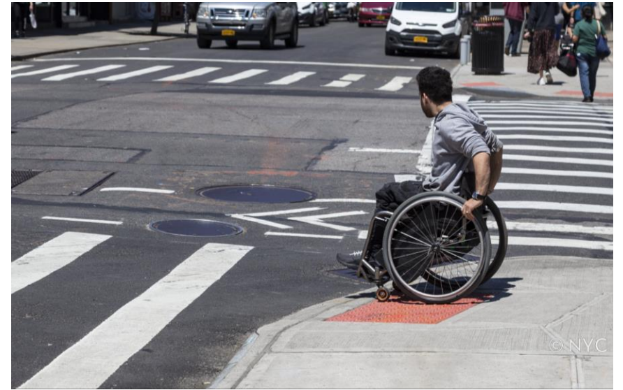
Pedestrian ramp ADA upgrades for improved accessibility
