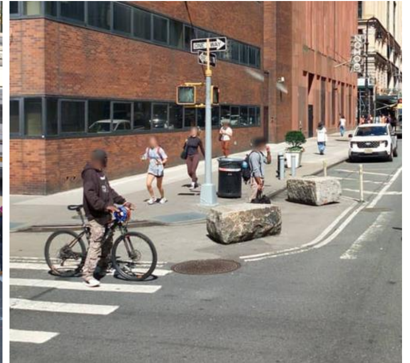
Proposed conditions (daylighting with painted curb extension and granite blocks) on select intersections (Photo: 4th St and Broadway, MN)
