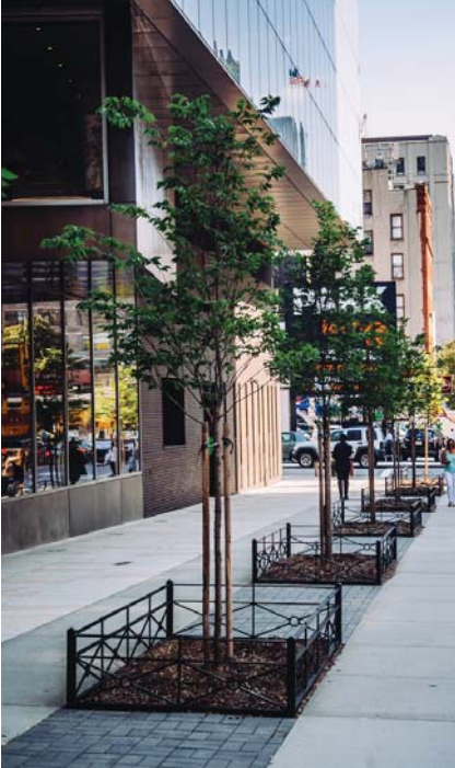
Permeable Pavers Usage: Health of Trees Provides space for stormwater and tree root growth
