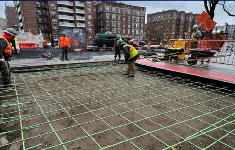
Grand Concourse Phase 4, currently under construction
