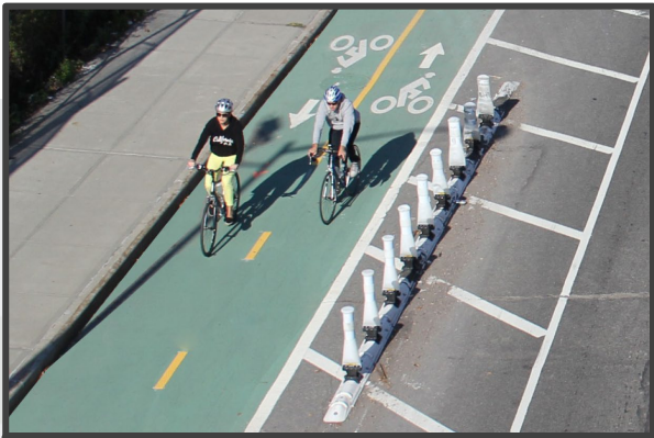
Quick Curb to Protect Cyclists
