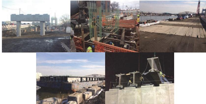
January 2017 – Mini Piles. February 2017 - Erection of the Concrete Beam – Timber Planks Over the Relieving Platform. Concrete Beams on Barge. (Credit: Artemio Angeles) Span 2.
