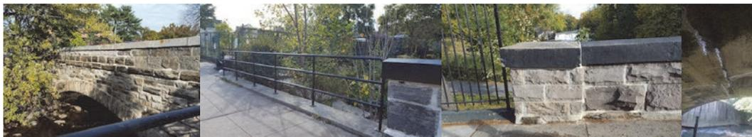
East 180<sup>th</sup> Street Bridge After Construction – South Wall, New Railing at South Sidewalk, North Parapet Wall, and Sealed Underdeck Cracks.
