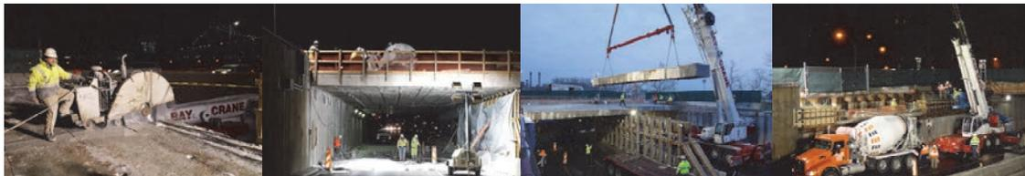
February 2017: Full Depth Saw Cutting of Deck Panels. Stage 3 - Protective Safety Shielding Over Highway. Loading of Deck Slab Panels for Disposal Off-Site. March 2017: Concrete Placement at West Abutment Wall Seat.
