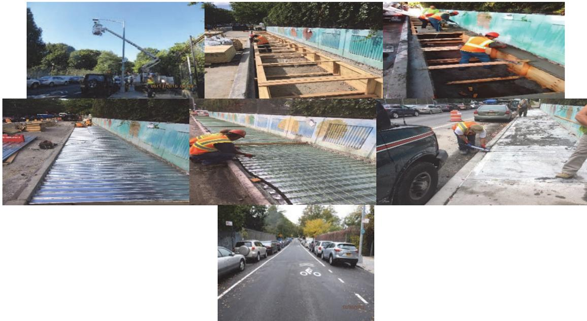
80<sup>th</sup> Road Bridge Under Construction. October 2017: End Approach Pavement and Spans 1 to 3 Wearing Surface Repaved With Asphalt Concrete. (October Credit: NYSDOT)
