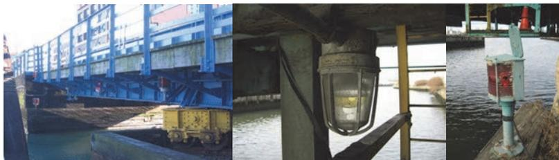
Inspection in Late 2012: Carroll Street Bridge - Navigational Fixtures on North Side of Span – Only the Center Span Fixture was Operational. Grand Street Bridge – Standing Water in the Access Light Fixture at the East Wedge Walkway. Typical Impact Damage to Pier Light.
