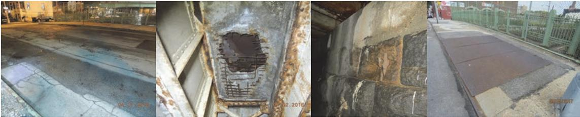
April 2016: Span 1, Wearing Surface at Mid-Span – Uneven Asphalt Patches on Approximately 40% of the Surface Area. Underdeck of Span 1- Through Hole and a Deep Spall With Exposed Rebar Near the End Abutment. There is a Steel Cover Plate Above. (April Credit: NYSDOT) February 2017: Beginning Abutment Masonry Stem Exhibits Missing Mortar Joint. September 2017: The 3 Steel Plates on the Left Sidewalk.
