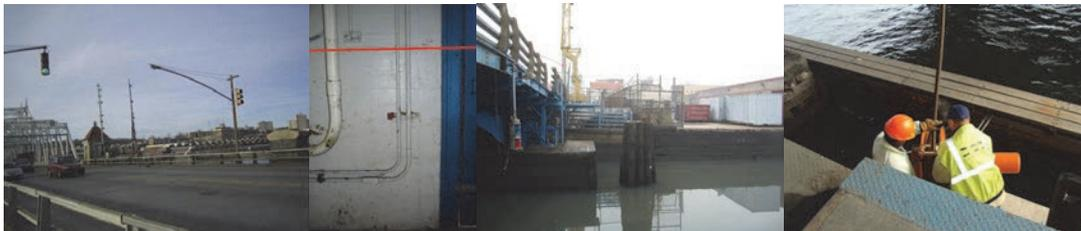
Inspection in Late 2012: East End of the West 207<sup>th</sup> Street Bridge - Missing Traffic Signal was Knocked Down by the Hurricane Winds. Borden Avenue Bridge Operator's House Basement Level – Depicted Flood Line was Approximately 5 Feet Above the Floor. Third Street Bridge – Northwest Channel Light Missing. Ninth Street Bridge – Manually Pulling the Cable Reel Because the Motor Failed.
