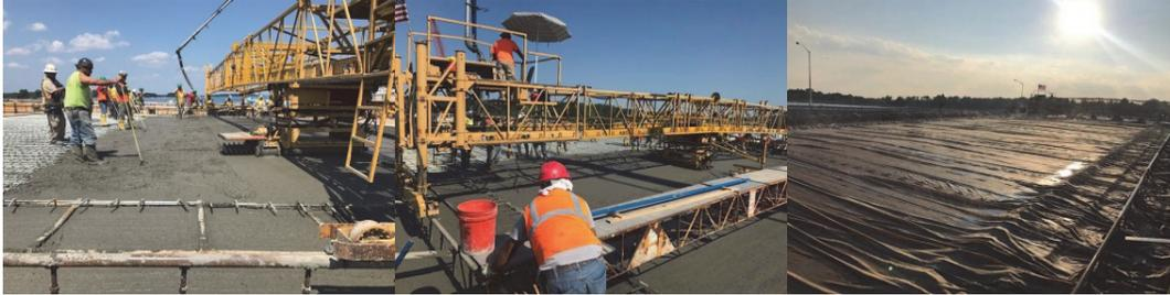
August 2017: Placing Concrete on the Deck Portion Near the East Abutment. A Finishing Machine Smoothing the Concrete Surface. A Wet Burlap and Soaking Hoses are Placed to Properly Cure the Deck.
