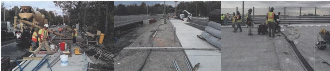
October 2017: West Approach Roadway – Placing Concrete at the North Approach. Installing Fencing Along the South Sidewalk. Bridge Deck – Completing the Installation of the Modular Joints.
