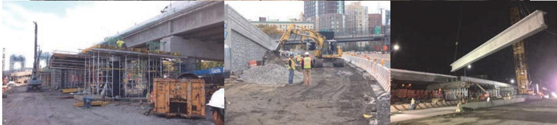
September 2017. October 2017: Enclosure to Protect the “Crack is Wack” Mural in the Park. Site View. Drainage Work at North Approach - Along Future Ramp D. November 2017: Last of the Pre-Stressed NEBT Girders for the Southbound Structure. (Credit: Artemio Angeles)
