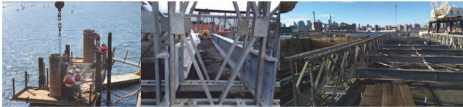
October 2014: The Contractor Airlifted Drilled Shaft Casings Into Position on a Platform Constructed Beside a Construction Barge. The Contractor Assembled the Temporary Bridge Segments at the Brooklyn Navy Yard. The Pieces Were Transported to City Island by Barge.
