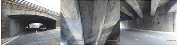
Douglaston Parkway Bridge Southbound Over Cross Island Parkway. March 2016: Right Elevation. Span 1 Concrete Beams Exhibit Spalls With Exposed Rebar Which Are Covered by Wire-Mesh Netting. (Credit: NYSDOT)
