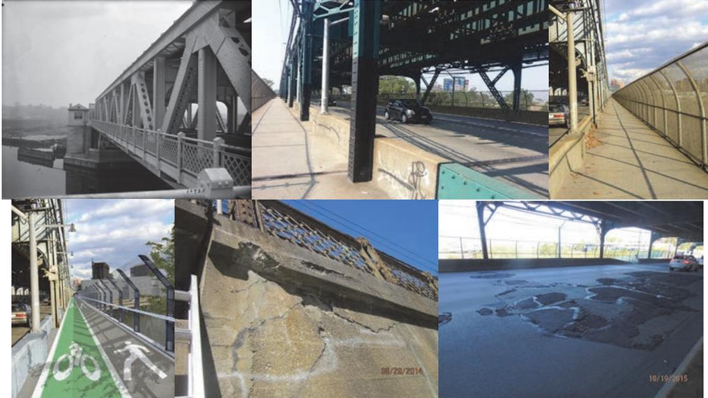
Roosevelt Avenue Bridge – In 1927. (Credit: NYC Records). Looking East. Existing and Proposed Bicycle/Pedestrian Path. 2014: Right Wingwall at the End Abutment. The Top Exhibits an area of Diagonal Cracks With Efflorescence and Spalls. The Deteriorated Concrete Areas are in Safe and Stable Condition. 2015: Spans 26 and 27 – Examples of Uneven Asphalt Patches and Broken Concrete Areas. (Credit: NYSDOT)
