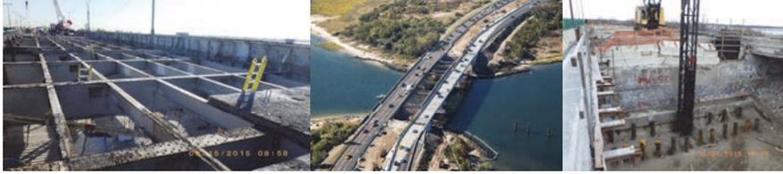
Deck Removed Prior to Steel Removal. October 2015: Stage 2 Traffic Pattern. Westbound Traffic at Right on New Bridge. Eastbound Traffic at Left on Existing Bridge. December 2015: Driving 14-Inch Diameter Steel Shell Piles at East Abutment - Facing East.
