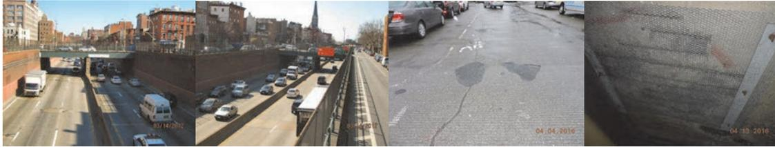
Sackett Street Bridge Over Brooklyn-Queens Expressway. March 2012: Elevation Left and Right. April 2016: Span 1 Wearing Surface. Span 2, Underside of Reinforced Concrete Deck Near the End Abutment - Exhibits a Spalled Area With Exposed and Corroded Rebars. This Location is Protected by Wire Mesh Netting. (Credit: NYSDOT)
