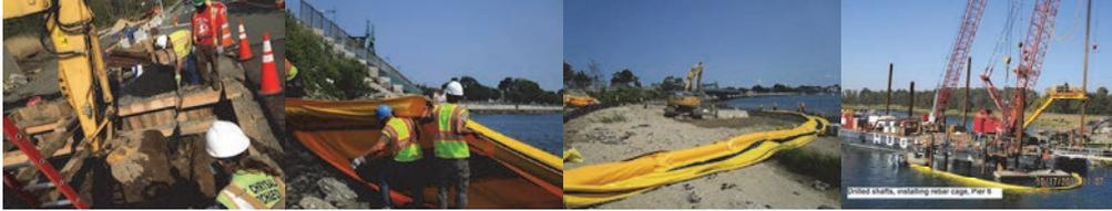
August 2014: Excavating on the West Side of the Bridge in the Presence of an Archeologist. Approximately 300 Linear Feet of a Turbidity Curtain was Installed on the Southwest Side of the Bridge to Protect the Shore During Construction. A Turbidity Curtain is a Floating Barrier Designed to Contain and Control the Dispersion of Sediment. October 2014: Drilled Shafts – Installing Rebar Cage at Pier 6.
