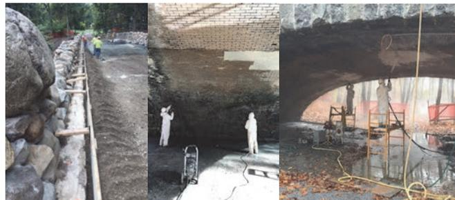
October 2016: Concrete Curb Layout. November 2016: Cleaning the Bricks Under the Bridge Arch. December 2016: Cleaning the Historic Stone Masonry and Removing Graffiti.
