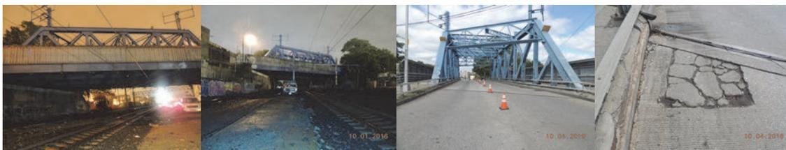
Unionport Road Bridge Over Amtrak – CSX. October 2016: Elevation Left and Right. Beginning Approach. End Approach, Top of Roadway at Right Truss- Exhibits a Spall and Joint Exhibits Torn Sealant. (Credit: NYSDOT)
