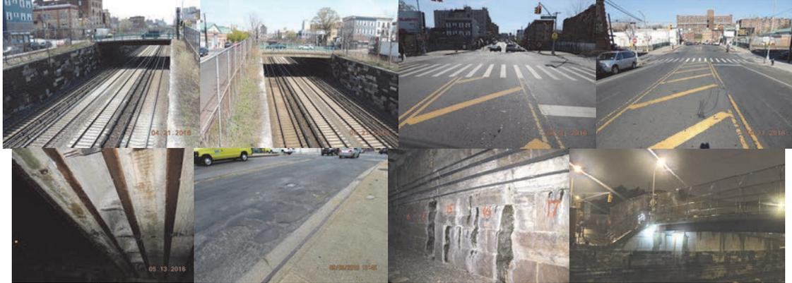
East 180<sup>th</sup> Street Bridge: April 2016 - Left and Right Elevations. Beginning and End Approaches. May 2016: Diaphragms in Bay 2 Exhibit Underside Spalling With Exposed, Debonded Rebar. (Credit: NYSDOT) September 2016: The Left Side of the Roadway Looking Toward the Beginning Abutment - The Wearing Surface Exhibits an Uneven Surface, Map Cracking and Small Potholes. February 2017: End Abutment Looking Northeast. Water Leakage Stains on the Bottom Portion of the Stem. Night View.
