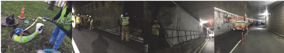
April 2016 - Installing Cables. July 2016: Painting Standpipe in the Southbound Battery Park Underpass. August 2016: Installing Conduits in the West Street Underpass.
