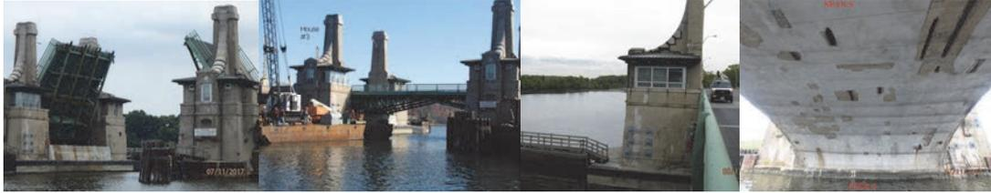
Bridge Open in July 2017. (Credit: NYSDOT) General View of Bridge Operator House #3 in 2011. Bridge Operator House #3 Exterior Wall in 2016, Looking Northwest. July 2017: Underside of Arch Span # 5 - Spalled Concrete With Exposed Rebar is Secured With Netting.
