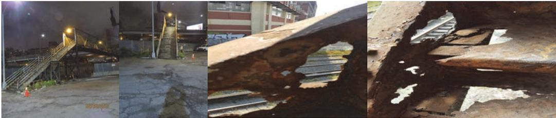
June 2017: Looking North at Spans 3-5, on Left Side - Staircase Stringers and Railing Exhibit Signs of Deteriorating Paint Throughout. End Approach, Looking Northeast – The Approach Wearing Surface Exhibits Spalls and Map Cracks Throughout. September 2017: Close-up View of Holes in Left Side Stringer, Steps and Risers.
