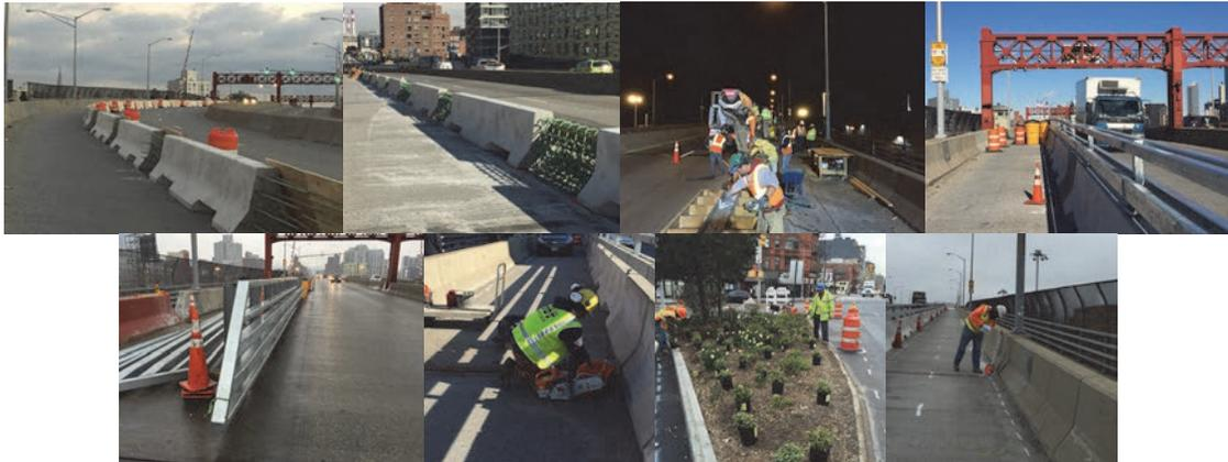
Pulaski Bridge - Precast Concrete Barrier in Place. Cast in Place Concrete Barrier Reinforcement. Cast in Place Concrete Placement. Two Rails Bicycle Railing. Five Rails Railing (Queens Flanking Span). Bridge Joint Seal Modification. Planting at Jackson Avenue Median. Layout for Roadway Striping.
