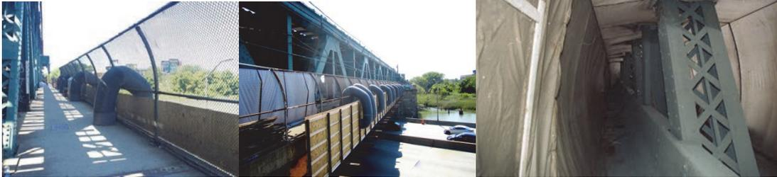
September 2016: - The Contractor Employs a Vacuum System to Capture Lead Particles During the Lead-Abatement Process. This is Done Using Negative Air Pressure to Prevent Emissions From the Abrasive Blasting Process Used to Remove Lead Paint. All Blasting is Done Within Negative Air Containment Units to Protect the Public From Emissions. View Inside the Containment – Bascule Span, Looking East.
