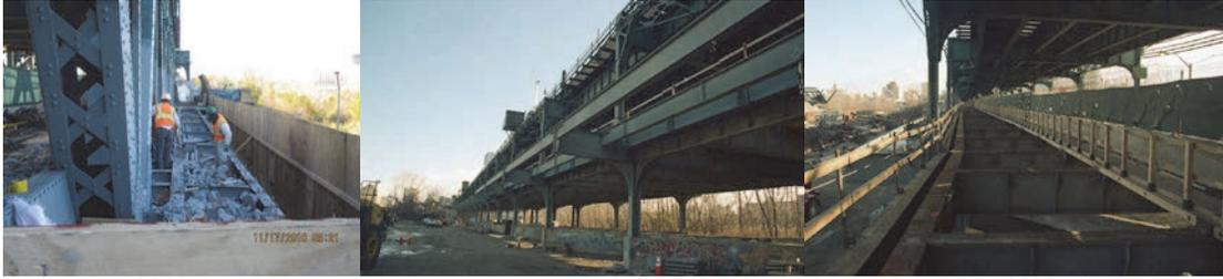
October 2016: Installing the New North Sidewalk – West Viaduct, Looking East. November 2016: Contractor Demolishes the Sidewalk over Van Wyck Expressway. East Viaduct – Stage 1 Installing the North Sidewalk Steel. December 2016: Installed North Sidewalk Stringers. West Viaduct – Roadway Deck Removed.
