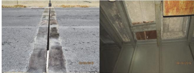
2016: Pier 102, Deck Joint at Southbound Roadway – Missing Joint Sealer Material. Span 143, Underside of Deck – Deep Spall. (Credit: NYSDOT)
