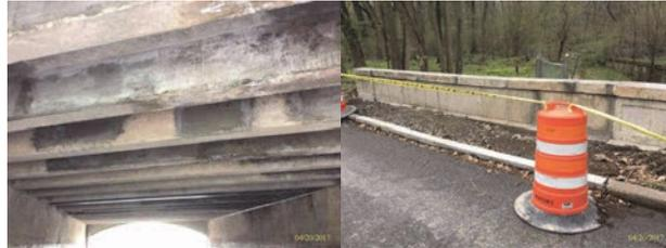
April 2017: Superstructure Framing – Repaired Concrete-Encased Steel Stringers and Concrete Underdeck. Begin Approach, Left Curb - New Segment of Concrete Curb. (Credit: NYSDOT)
