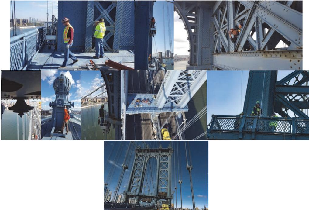
Ornaments on the Manhattan Bridge Towers Were Flagged as Potentially Hazardous and Removed by In-House Ironworkers in October and November 2016. (Credit: Bojidar Yanev) Using Spider to Remove Ornament at Cable C West in 2016. (Credit: Samuel Teaw)
