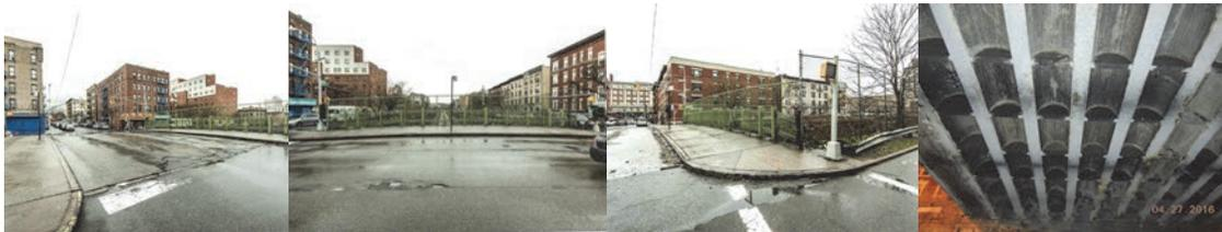
East 187<sup>th</sup> Street Bridge over Metro North Before Construction - Southeast and North Views. Southwest Crosswalk. April 2016: Span 1, Underside of Deck Exhibited Minor Mapcracking and Efflorescence. (Credit: NYSDOT)
