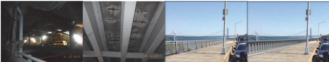
2015: Underside of Span 30, Looking Southwest (NYCDOT Maintenance Garage Area). 2017: Span 5 Underside of Deck Bays 16 and 17 - Spalls With Exposed Rebars. (Credit: NYSDOT) Current and Proposed Bridge Railing.
