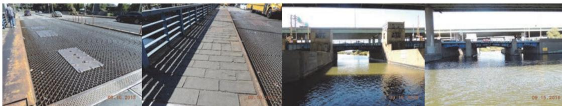
2015: Span #9, Open Deck Grating at Westbound Roadway, Looking Ahead and Right. Loose and Bouncing Plates. Plastic Delineator Posts Mounted to the Concrete Median are Missing the Majority of Posts Due to Vehicular Impacts. Span #9 Right Sidewalk, Looking Back. Asphalt Tiles Over the Bascule Span are Severely Deteriorated and Exhibit Several Missing Tiles. Existing Bridge in September 2016 – Left and Right Elevations. (Credit: NYSDOT)
