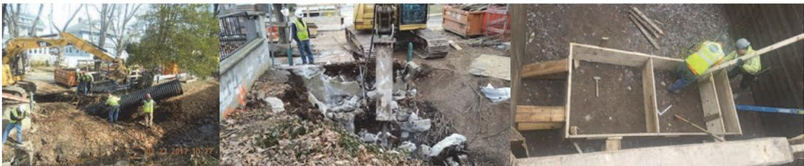
Gregg Place Culvert in February 2017. Looking Northeast - Installation of 30 Inch Pipe for Water Diversion Structure. March 2017 - Looking South - Forming up Footings for the Headwall.
