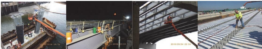
July 2016: Pier #2. Placing Pier Column Forms Around Galvanized Steel Rebar Cages on Top of Plinth. August 2016: Placing High-Strength Bolts Through Girder Splice Plates. September 2016: Torqueing Girder Web Splice Plate Bolts. October 2016: Welder Attaching Shear Studs to the Top Flange of the Eastbound Bridge During Stage 2.
