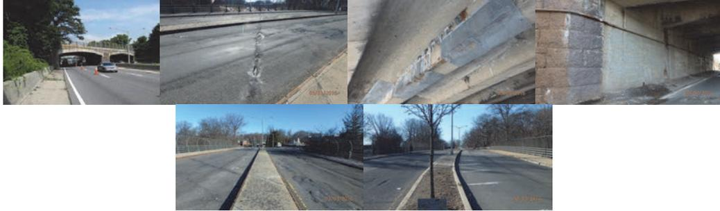
Douglaston Parkway Bridge Northbound Over Cross Island Parkway. March 2016: Top of Bridge, Asphalt Wearing Surface Above Beginning Abutment - Spalls and Uneven Wearing Surface. Span 1 - Deteriorated Concrete Covered With Wire Mesh. Abutment End. Approach Begin and End. (Credit: NYSDOT)
