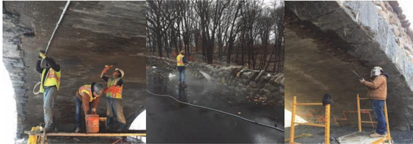
January 2017: Tuck Pointing the Bricks. Power Washing the North Parapet Wall.
