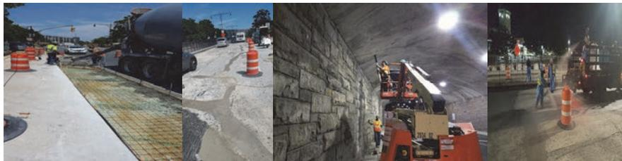
Southern Boulevard Bridge During Construction – Sidewalk Repair, Deck Repair, Weep Hole Installation, and Waterproofing.
