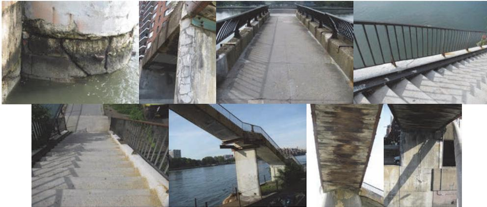
Bridge Conditions in June 2014. Pier 1 Over the East River – Close-up of 2 Wide Cracks. Begin Abutment Stem Right Side - Failing Patch and Map Cracking. Span 1 Deck Wearing Surface. Span 2 Railing. Span 3 Concrete Steps. Pier 2, Under Span 2, Looking Southwest – Spalled Concrete Area With Exposed Rebar at Bottom of Pier. Underdeck of Span 1. Begin Abutment Stem.
