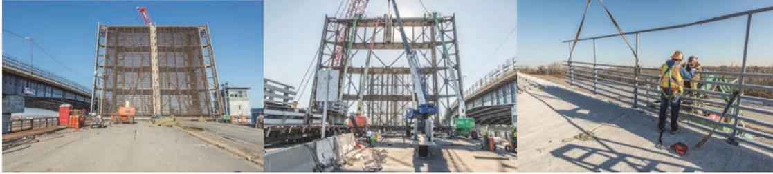
December 2017: South Leaf of the Mill Basin Bridge During Demolition. Sidewalk and Median Removed. The New Bridge is at Left Carrying Eastbound and Westbound Belt Parkway Traffic. North Leaf of the Mill Basin Bridge During Demolition. Steel Bridge Deck, Median, and Walkways are Removed. New Mill Basin Bridge is at the Right Side. Erecting the 7-rail Bridge Rail and Fence at the East Side of the Bridge for the Bicycle/Pedestrian Walkway.
