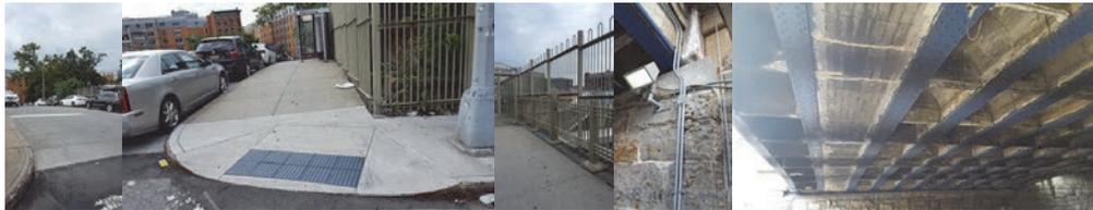
East 162<sup>nd</sup> Street Bridge After Construction – New Concrete Overlay. New Southwest Pedestrian Crossing. Repaired Pedestals. Painted Fence and Railing. Sealed Underdeck Cracks.
