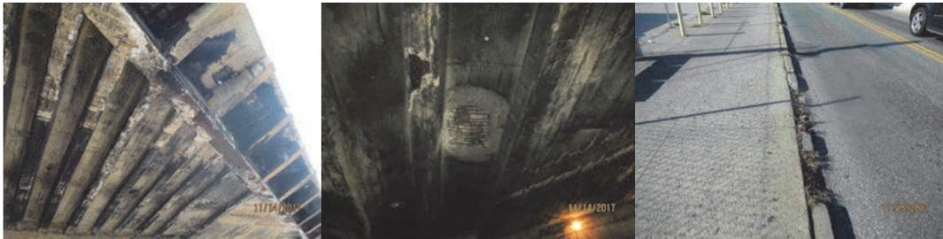
Span 2, Underside of Deck- Spalled Concrete Encasement and Deck. Exposed Rebar. Span 2, Top of Deck - Spalled and Missing Sections of Curb With Vegetation Growth. (Credit: NYSDOT)
