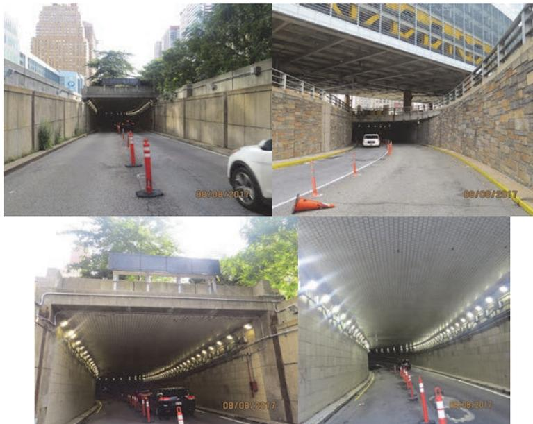
August 2017: West Street Underpass Elevation North and South. North Concrete Portal. Variable Message Board Will Be Replaced.
