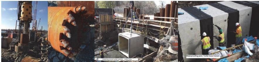
January 2015: Drilling Rig Construction Vehicle Used to Install Land-Based Drilled Shaft Casing for the Temporary Bridge. The Bucket Drills Carve Out the Casings With Teeth Capable of Tearing Through Rock. April 2015: Turtle Cove Culvert Replacement. Installing Culvert Under the Utilities. May 2015: Waterproofing the Joint.
