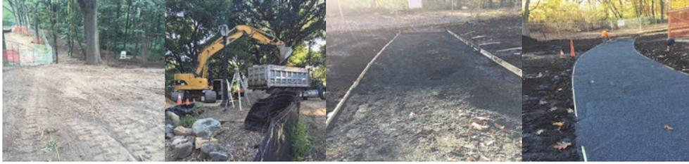
August 2016: North and South of Bridge – Clearing and Grubbing. November 2016 Placing Granular Fill Material (Crushed Stone) on the Bridge Pathway Under the Bridge Arch.
