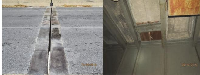
2016: Pier 102, Deck Joint at Southbound Roadway – Missing Joint Sealer Material. Span 143, Underside of Deck – Deep Spall. (Credit: NYSDOT)
