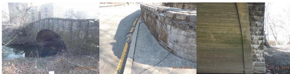
Bronx Boulevard Southbound Bridge Over Bronx River. March 2012: Elevation Left Span. March 2016: Span 1, Right Parapet - Exhibits Spall With a Full Height Vertical Crack. Span 1 – Efflorescence on Underside of Stone Masonry. (Credit: NYSDOT)
