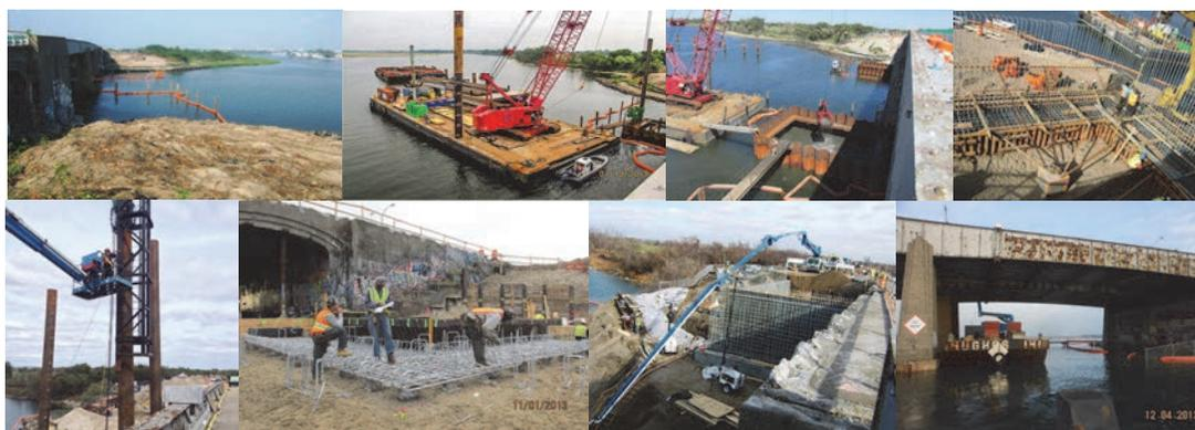
June 2013: North Side of Gerritsen Bridge - Turbidity Curtains Placed on Both Sides of Navigable Channel. July 2013: Work Barges Driving Steel Sheeting for Pier #1 Cofferdam. September 2013: Rebars and Form Work for Footing and Walls at the Northwest Abutment. Stage 1 Piles. October 2013: Inspecting Rebar. November 2013: Tremie Concrete Pour at Pier #2. December 2013: Inspecting Spans 7 and 8 of the Existing Bridge From a Barge. (Inspection Credit: NYSDOT)
