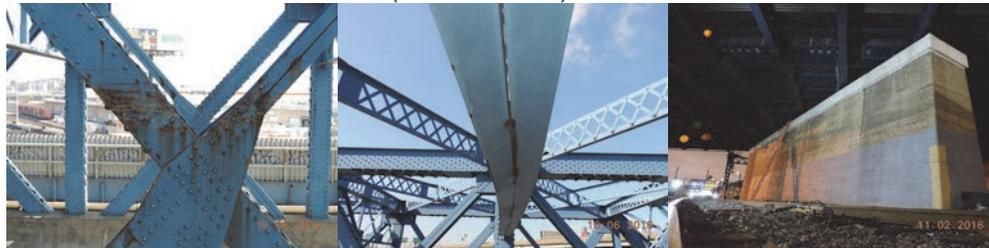
Span 2, Truss T2 - Left Face of the Gusset Plate and Adjacent Diagonal Member Exhibit Scrape Marks and Paint Loss With Minor Surface Corrosion Due to Vehicular Impact. Span 1, Sway Strut Bracing Between Truss T2 and T3 - Brace Bottom Flange Exhibits Bending Toward Span 2 due to Vehicular Impact. Pier 1. (Credit: NYSDOT)
