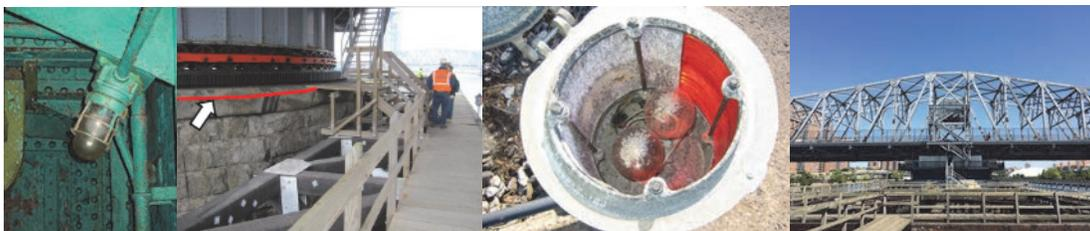
Inspection in Late 2012: Union Street Bridge – Standing Water in East Span Maintenance Light. Madison Avenue Bridge - General View of Fender and Center Pier—the Red Line Depicts the Approximate Water Level. Macombs Dam Bridge – Pier Lighting Fixture with Cover Removed – Silt Deposit on Lamp Tops, and Corrosion on the Fixture Frame. 145<sup>th</sup> Street Bridge in August 2015. (Credit: Lity Barreto)
