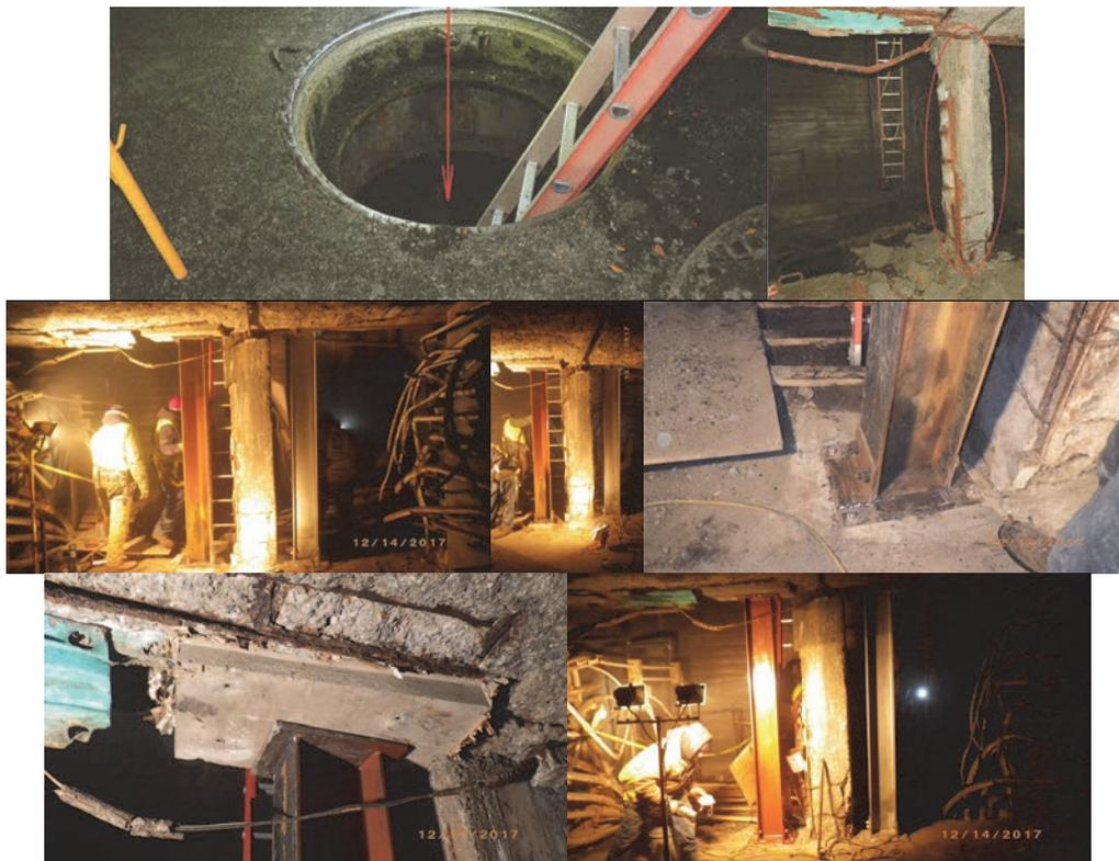
Entrance to the Confined Space. Span 34, Spalled Support Column with Exposed Main Rebars and Broken Stirrups.
