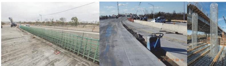
Mill Basin October 2017: Epoxy Coated Rebars for Future Left Side Barrier of Westbound Mill Basin Bridge. The Westbound Traffic is on the Eastbound Side of the New Bridge in This Stage. November 2017: Belt Parkway Roadway Facing South. Westbound Traffic on the Right Side Going Over the New Mill Basin Bridge. Left Side Shows New Roadway Prior to the Shift of Eastbound Traffic onto the New Bridge.
