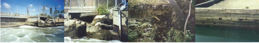
From Study of the FDR Drive: Location #2 – Damaged Seawall at Segment #5. Sinkhole at Location #6 at East 59<sup>th</sup> Street. From Study of Carroll Street Bridge: General View of the Southwest Crib Wall With the Delamination of the Timber Stretchers in the Tidal Zone.
