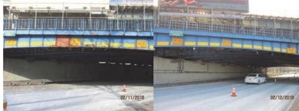
2016: Span 1 Right Sidewalk Near Beginning Abutment – Steel Plates. Girder Reinforced With New Steel Plate and Angles. Strongback Girder at Right Side of Span 1. Right and Left Fascia. (Credit: NYSDOT)
