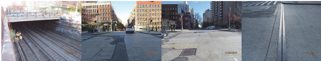
East 97<sup>th</sup> Street Bridge over Metro North. 2016: Beginning and Ending Approaches. Beginning Abutment Joint - Deteriorated Sealer Material. (Credit: NYSDOT)
