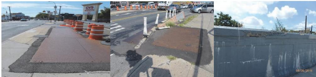
August 2016: Span 2 Left Sidewalk Looking South - Location of the Through Hole. Span 1 Right Sidewalk Looking North. Spalled and Cracked Areas on Top of Span 2 Parapet. (Parapet Credit: NYSDOT)
