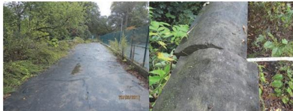
Hill Drive Bridge in 2017: Spans 1 Through 3, Asphalt Wearing Surface - The Deck Top Exhibits Large Areas of Cracked Pavement Due to Deck Deterioration Along the Entire Left Side of the Bridge for a Width of Approximately 12 feet. Most of These Cracks Have Been Sealed With Bituminous Material. Water Seeping Through These Sealed Cracks is Causing Heavy Deterioration of the Deck. Span 1, Stone Coping on Left Railing. (Credit: NYSDOT)
