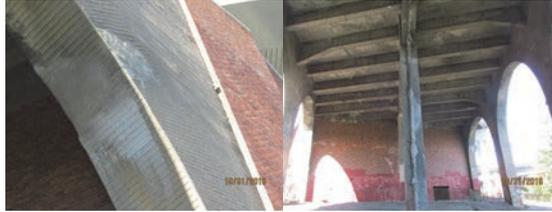
October 2016: Span 51, Underside of Right Arch - Concrete Repairs. Pier 49, at Center Column - Concrete Repairs.
