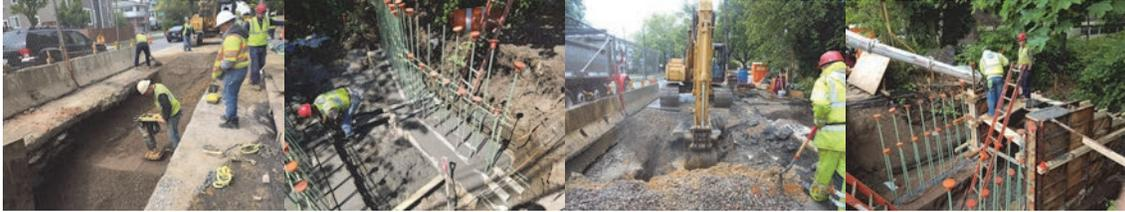
Forest Avenue Culvert over Randall Avenue in May 2017 - Looking West. Backfilling the Trench Over the New 20 Inch Iron Pipe Water Main. Looking South - Placing Rebar for Wingwall Footing. Looking West - Excavating and Removing the Old Culvert. Looking Northwest. Placing Concrete Into Formwork for the Wingwalls.
