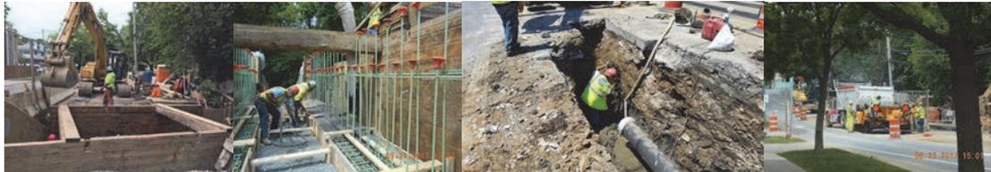
May 2017 - Looking West - Installing Shoring Around Excavation. Looking North - Placing Concrete for Footing. June 2017 - . Looking Down and Northwest Along Forest Avenue - Installing the New 12 Inch Water Main. Looking Northwest - Placing Temporary Asphalt Over 12 Inch Water Main Trench on Forest Avenue.
