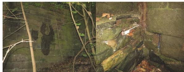
Hill Drive Bridge in 2017: Span 1, Left Exterior Enclosed Wall. End Abutment, Stones on Left Wingwall – Void Due to Missing Stones. . (Credit: NYSDOT)
