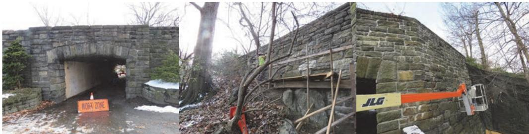
December 2017: Maintenance Workers Adding Mortar to the Joints on the Beginning and Ending Right Side Wing Walls of the Margaret Corbin Drive Bridge over Pedestrian Path Near the North Entrance.
