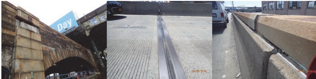
May 2016: Span 43, Right Side Fascia - the Stone Masonry Curtain Wall Exhibits Localized Moderate to Heavy Efflorescence Formation at Several Mortar Joints at the Outside Face and at the Underside of the Arch. Pier 19 Joint, Atlantic Avenue Westbound - Approximately 40% Length of Joint Compression Seal is Slightly Debonded. Spans 33 thru 35, Top of Deck, Right Fascia at Right Bridge Railing - Separation (up to 2") of the Fascia Stones From the Bridge Railing. (Credit: NYSDOT)
