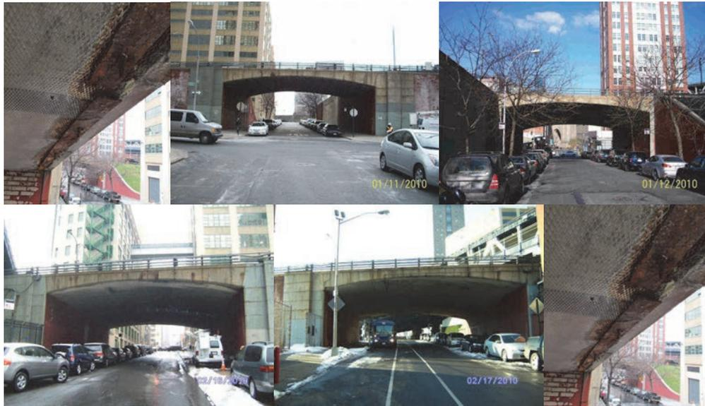
In general, the arch bridges have an adequate load-carrying capacity, however, there are areas of map cracking and visible leakage through the joints. Mesh has been installed at the underside of the deck to prevent debris from falling on vehicles or pedestrians below.
