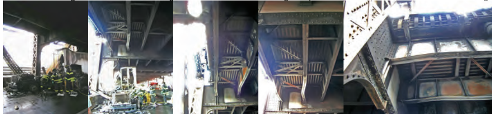
September 2008: Advanced Corrosion of Steel Stringer and Girder. February 2011: Red Flag Stringer Repair at Riverside Drive Viaduct over West 158 th Street. July 2015: Assistant Civil Engineers Andrew Hoang and Clara Medina Inspecting a Red Flag on the Manhattan Bridge From the Motorized Bridge Inspection Traveler Platform Beneath the Bridge.
