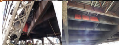
August 2013 Red Flags on the Ed Koch Queensboro Bridge. October 2013: Removing the Warped Beams. The New Beams.
