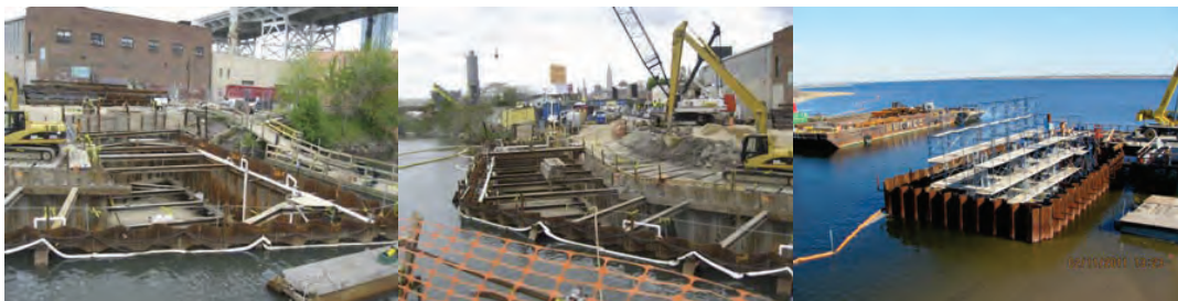
April 2010: Cofferdam With Filter Fabric and Gravel Placed Prior to Pile Driving During the Emergency Repair Project on the Borden Avenue Bridge over Dutch Kills. February 2011: Fresh Creek Cofferdam Pad.
