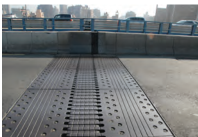
Manhattan Bridge Finger Dam. (Credit: Jagtar Khinda)
