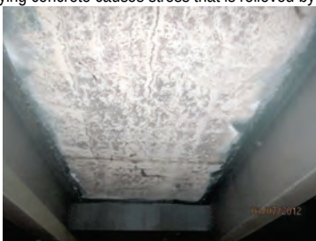
Union Street Bridge over Brooklyn-Queens Expressway in 2012 – Extensive Map Cracking With Efflorescence on the Underside of the Deck. (Credit: NYSDOT)
