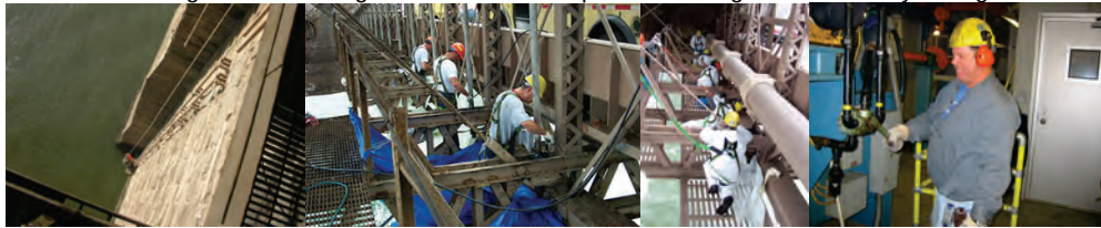
Repairing the Brooklyn Bridge Standpipe System, 130 Feet Below the Roadway. Maintenance Crew Conducting the Annual Cleaning and Lubrication of the Solid Rod Suspenders and Spherical Bearings on the Brooklyn Bridge. 2 nd Photo - Oilers Steven Marxhausen, Rene Francis, Richard Morreale, Thomas McAuliffe, and Andrew Sorrentino. (Credit: Anatoly Orlov) Oiler T. McAuliffe at the 9 th Street Bridge
