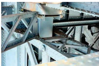
Truss Bearing on Manhattan Bridge. (Credit: NYSDOT)
