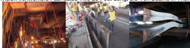
August 2013 Red Flags on the Ed Koch Queensboro Bridge. A truck caught fire on the bridge and damaged three stringers that support the eastbound upper roadway. Replacement of the two damaged stringers and the repair of a third were completed in October 2013. All work was performed by in-house forces. August 2013: Firefighters Examining the Damage. Repairing the Bridge Included Custom Designing the Steel Beams, as Well as Fabrication and Installation. Division Ironworkers Fabricated Two 26-Foot-Long, 1.5-Ton Beams in Their Brooklyn Shop.
