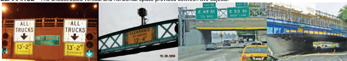
United Nations – 1 st Avenue Tunnel Vertical Clearance Posting. Grand Street Vertical Clearance Posting. (Credit: NYSDOT) Retro-reflective Material Improves Visibility of These Low Vertical Clearance Bridges: East 60 th Street Bridge Over FDR Drive and Westchester Avenue Bridge over Hutchinson River Parkway.
