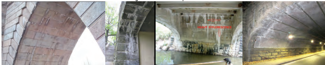
Moderate Efflorescence on the Brooklyn Bridge Brooklyn Tower North Gothic Arch in 2004. (Credit: NYSDOT) Efflorescence on the Underside of the Masonry Stones on the End Abutment of the Margaret Corbin Drive Bridge over Pedestrian Path Near Café. Heavy Efflorescence on End Abutment Stem Wall of Bridge Over Dam at Clove Lake in 2014. Efflorescent Stains on the Shielding of Span #1 of the East Drive Bridge over Transverse Road #3 in 2015.
