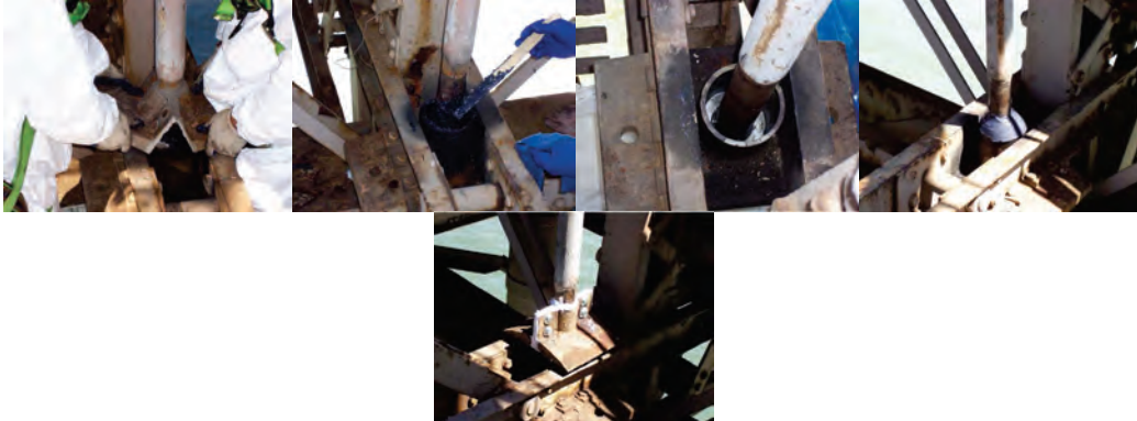
Cleaning and Lubricating the Solid Rods' Suspender Bearings on the Brooklyn Bridge.
