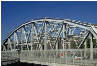
Macombs Dam Camelback Truss.
