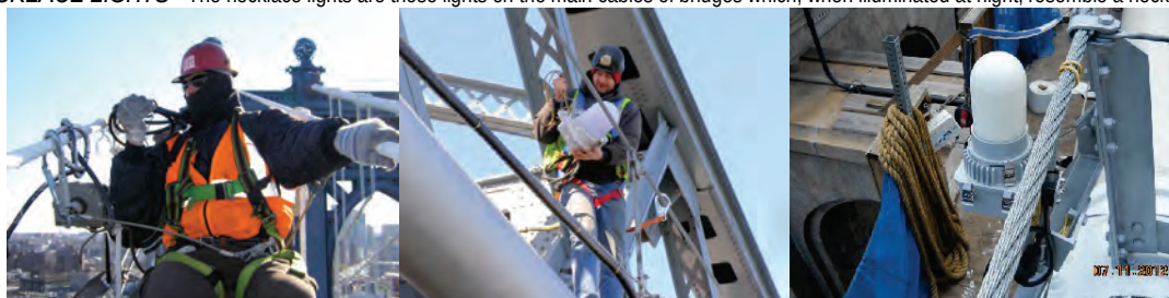
Repairing a Manhattan Bridge Necklight. Bridge Repairer and Riveter Neil Dalton Installing a New Light on the Williamsburg Bridge in 2012. (Credit: Hany Soliman) Manhattan Bridge Side Necklight. (Credit: NYSDOT)
