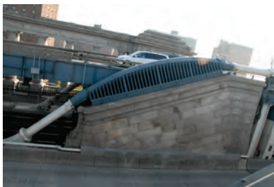
Manhattan Bridge Saddle. (Credit: Jagtar Khinda)
