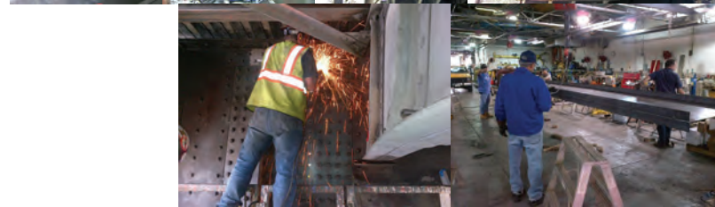
August 2013 Red Flags on the Ed Koch Queensboro Bridge. A truck caught fire on the bridge and damaged three stringers that support the eastbound upper roadway. Replacement of the two damaged stringers and the repair of a third were completed in October 2013. All work was performed by in-house forces. August 2013: Firefighters Examining the Damage. Repairing the Bridge Included Custom Designing the Steel Beams, as Well as Fabrication and Installation. Division Ironworkers Fabricated Two 26-Foot-Long, 1.5-Ton Beams in Their Brooklyn Shop.
