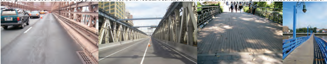
Brooklyn Bridge Wearing Surface. Manhattan Bridge Wearing Surface and Safety-Shaped Barriers. (Credit: NYSDOT) West 86 th Street Pedestrian Bridge (Southwest Reservoir Bridge) Wooden Wearing Surface. Ocean Avenue Pedestrian Bridge over Sheepshead Bay.
