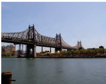
Ed Koch Queensboro Bridge (Credit: Russell Holcomb)
