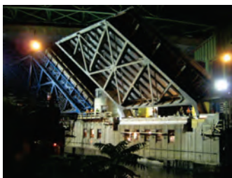
Leaves of the Hamilton Avenue Bridge.
