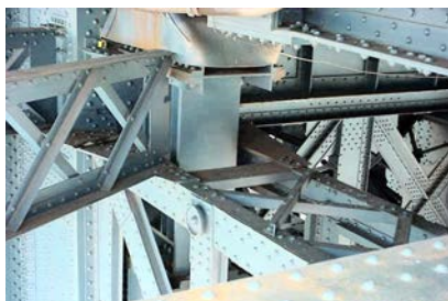
Truss Bearing on Manhattan Bridge. (Credit: NYSDOT)
