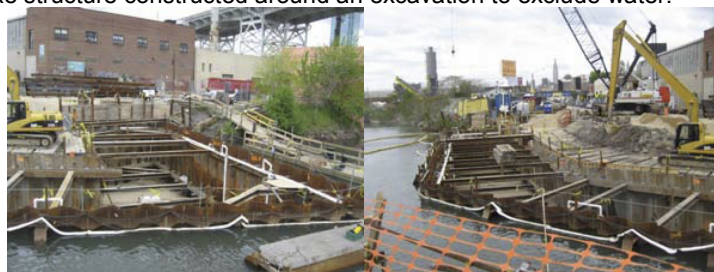
April 2010: Cofferdam With Filter Fabric and Gravel Placed Prior to Pile Driving During the Emergency Repair Project on the Borden Avenue Bridge over Dutch Kills.
