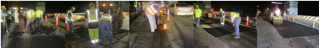
Resurfacing the Belt Parkway Bridge over Mill Basin on August 3, 2009. The Crew Completed a 13'x29' Cut in the Eastbound Center Lane, West Approach Spans. The Area Exhibited Rutting, Cracking and Excessive Patching. Breakout and Removal of Deteriorated Wearing Surface. Ironworker Assisting the Crew. Installation of New Asphalt. (Credit: Yousef Demis) Compacting the Asphalt With the Assistance of a Gasoline Roller Engineer From the Roadway Repair and Maintenance Division. (Credit: Ali Mozaffari)
