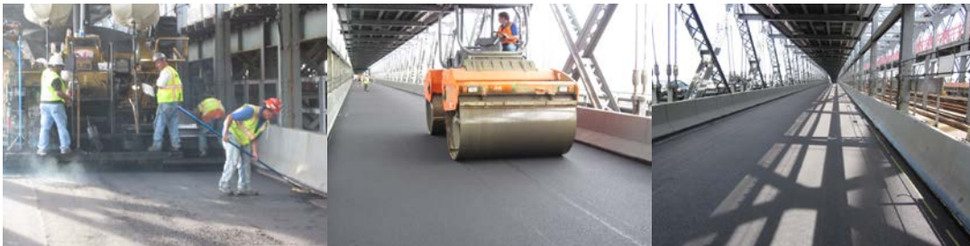
Repaving the Williamsburg Bridge in 2011.
