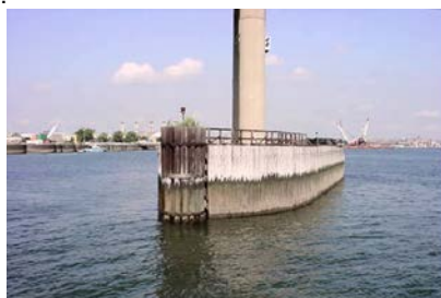
Rikers Island Dolphin & Fender System. (Credit: NYSDOT)
