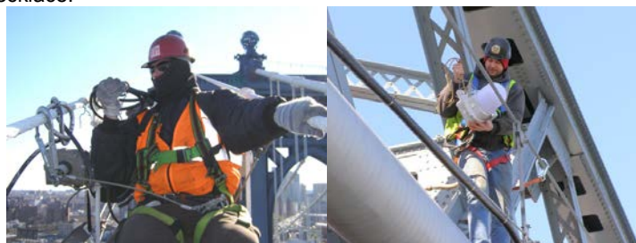
Repairing a Manhattan Bridge Necklace Light. Bridge Repairer and Riveter Neil Dalton Installing a New Light on the Williamsburg Bridge in 2012. (Credit: Hany Soliman)
