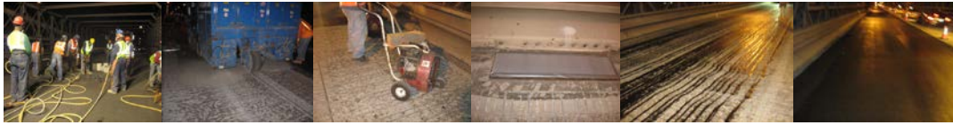
Removing the Old Micro-Surfacing on the In-Bound Brooklyn Bridge. Shot Blasting for Surface Preparation. Cleaning the Roadway Surface. (Credit: Fouad Althaibani, Emad Shaker, and Sunil Desai) 2008: Covering all the Drainage Systems Before Applying the Micro-Surfacing on the In-Bound Brooklyn Bridge. Applying the Tack Coat for the Micro-Surfacing. Applying the New Micro-Surfacing Materials. (Credit: Fouad Althaibani, Emad Shaker, and Sunil Desai)
