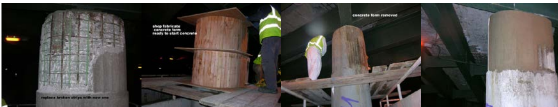
December 2013 – Repairing Deteriorated and Spalled Concrete (Yellow Flag) at the Top Portions of the Pier Columns on the Astoria Boulevard Bridge over BQE West Leg.
