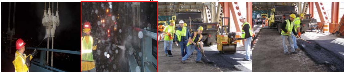
Power Washing the Corrosive Deicing Solvents Within the Range of the Roadway Splash Zone on The Manhattan Bridge in October 2007. Particular Attention is Directed to Cleaning the Gusset Plate. (Credit: Albert Hong)
