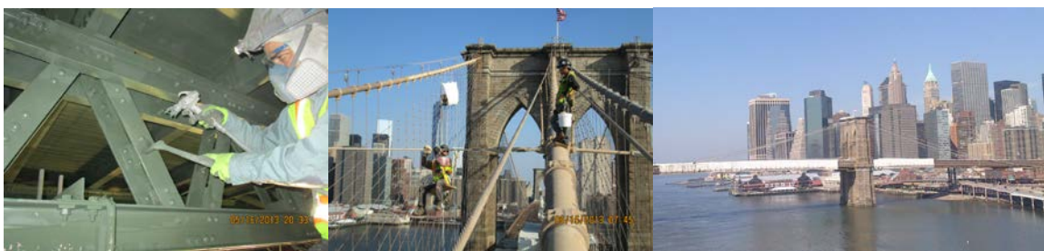
May 2013: Painter Applying Primer Stripe Coat on the Manhattan Main Span. June 2013: Painter on Sway Bracing on the Brooklyn Side Span. (View Credit: Earlene Powell)
