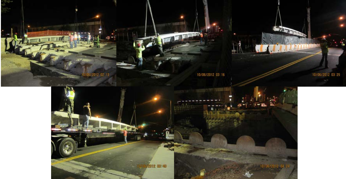
October 2012: Second Stage Demolition: Removal of the Remaining Portion (10 Concrete-Encased Steel Girders) of the Existing Bridge Superstructure.
