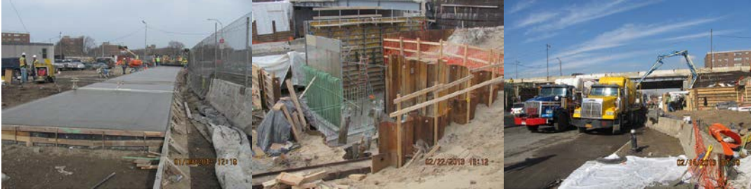
Rockaway Parkway Bridge in January 2013: Placing On-Grade Concrete Pavement at Ramp "D" Eastbound Entrance to the Belt Parkway. February 2013: Southeast Abutment Area Showing Steel Sheeting, Cast-in-Place Concrete-Filled Steel Pipe Piles, and Concrete Footing With Epoxy Coated Rebars. East Abutment Concreting.
