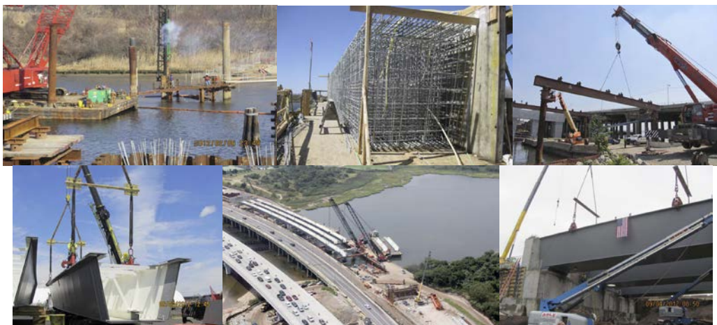
Paerdegat Basin Bridge in February 2012: Driving Piles for Temporary Work Trestles on the North Side for the Future Westbound Bridge. April 2012: Galvanized Steel Rebars for Westbound Pier 1 Cap Beam. June 2012: Erecting Steel Falsework Temporary Supports for the Westbound Paerdegat Tub Girders. Unloading Tub Girder Section for Westbound Paerdegat Basin Bridge at Contractor's Storage Yard. August 2012: Paerdegat Basin- Eastbound Belt Parkway Traffic on New Eastbound Bridge Shown at Left. Westbound Belt Parkway Traffic on Old Paerdegat Basin Bridge at Center. Tub Girder Erection in Progress at Right Side by Crane on a Temporary Work Platform at Future Westbound Bridge. September 2012: Setting the Last Tub Girder Section for the Westbound Bridge at the East Abutment.
