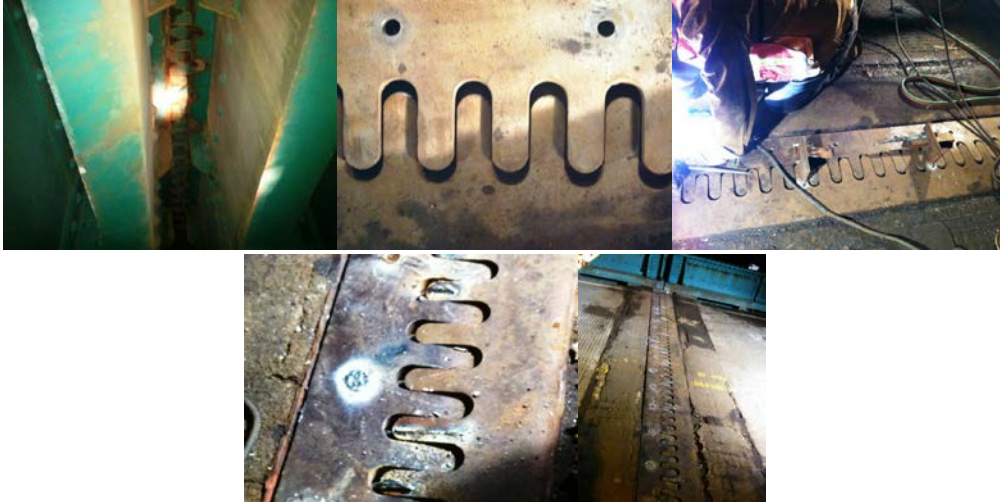
City Island Bridge: View Beneath the Finger Joint. The Joint Plates are Placed to Check for the Proper Gap. Leveling the Plate Before Welding. Close-Up of a Plug Weld. After 17 Plug Welds, the Finger Joints Sit Flush on the Roadway.
