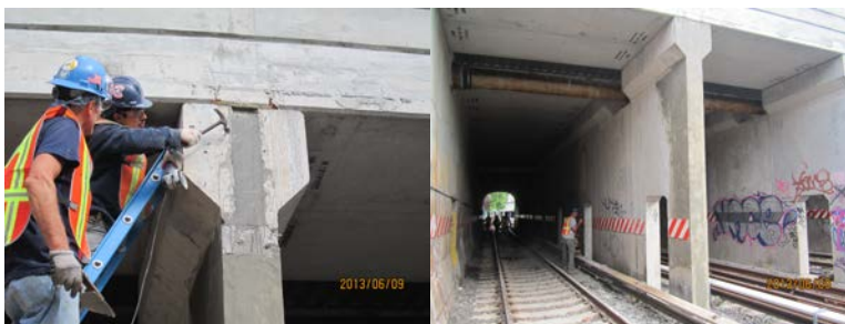
Removing Form Nails From the Stripped Keyway. The Completed Repairs.
