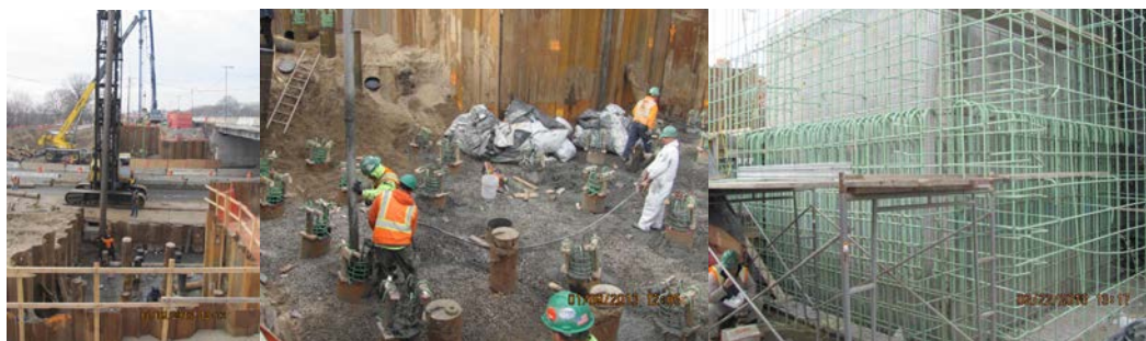
Rockaway Parkway Bridge in January 2013: Driving Steel Pipe Piles at the South East Abutment. Pumping and Vibrating Concrete into Steel Pipe Piles at the Southwest Abutment. Southwest Abutment Epoxy Coated Rebars for the Abutment Walls.
