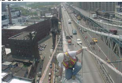
Inspector on Manhattan Bridge Cable. (Credit: NYSDOT)
