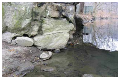
Scour on Pier 2 End Face of Moshulu Parkway Bridge Over Bronx River in 2008. (Credit: NYSDOT)
