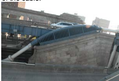
Manhattan Bridge Saddle. (Credit: Jagtar Khinda)
