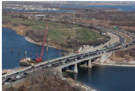
Gerritsen Bridge Facing North (Eastbound) - Driving Piles at Pier #2.
