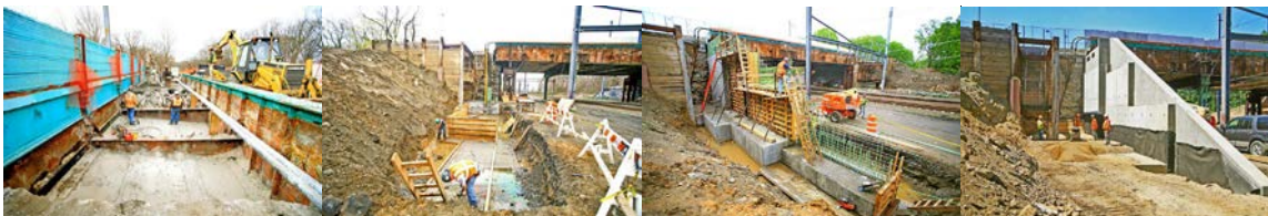
December 2010: Demolition of Existing Stage-1A Deck. April and May 2011: Formwork for Stage-1 Abutment Footing and Abutment. July 2011: Backfill Behind New Stage-1 Abutment.
