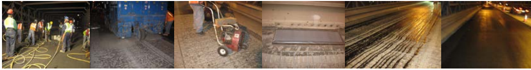
Removing the Old Micro-Surfacing on the In-Bound Brooklyn Bridge. Shot Blasting for Surface Preparation. Cleaning the Roadway Surface. (Credit: Fouad Althaibani, Emad Shaker, and Sunil Desai) 2008: Covering all the Drainage Systems Before Applying the Micro-Surfacing on the In-Bound Brooklyn Bridge. Applying the Tack Coat for the Micro-Surfacing. Applying the New Micro-Surfacing Materials. (Credit: Fouad Althaibani, Emad Shaker, and Sunil Desai)
