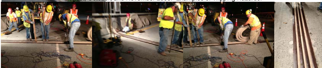
July 2013 Safety Flag: Ironworker and Mason Crews Repairing Missing Joint Seal Materials on the Brooklyn-Bound Williamsburg Bridge. The Joint Sealer Spaces Were Widened on Each Part of the Joint Utilizing the Shop-Made Jack Expansion Blocks, and Then Completely Cleaned With a Needle Gun to Prepare the Surface to be Rough Contacted With Epoxy Glue. After the Glue was Spread on the Sealer Space Surfaces, the Seal Strip was Installed and Tightened. (Credit: Hany Soliman)
