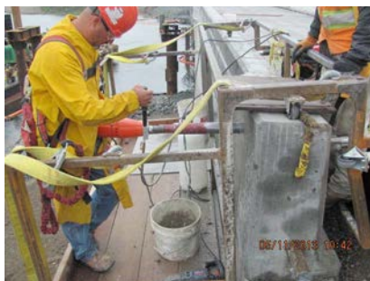
Drilling Through the Back of the Barrier to Install Box Beam Rail on the Face of the Barrier.
