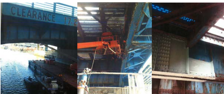
Bruckner Expressway Service Road Bridge over Westchester Creek (Unionport Bridge): Steel Repairs. Completed Steel Repair With Primer Paint Coat.
