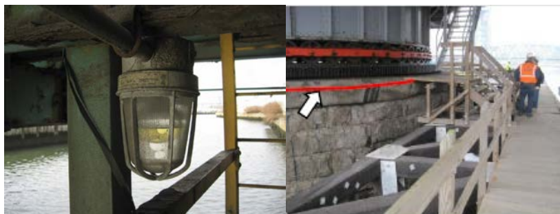
Grand Street Bridge – Standing Water in the Access Light Fixture at the East Wedge Walkway. Madison Avenue Bridge - General View of Fender and Center Pier—the Red Line Depicts the Approximate Water Level.
