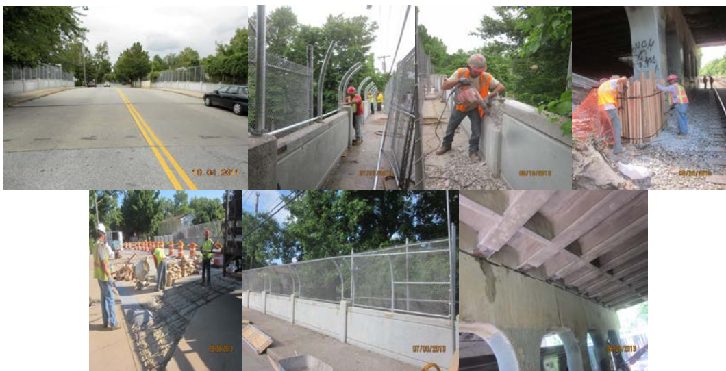
Albee Avenue Bridge. Repairing Fence and Fence Post, Pier Bent, and Deck Concrete. Bridge After Repair.
