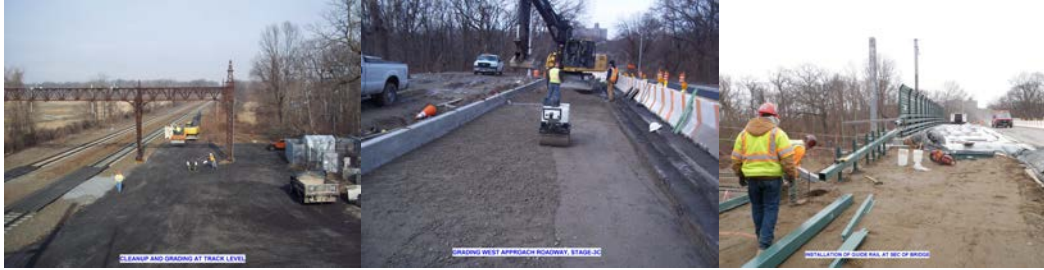
January 2013: Cleanup And Grading at Track Level. Stage 3C: Grading West Approach. Installing Guide Rail.
