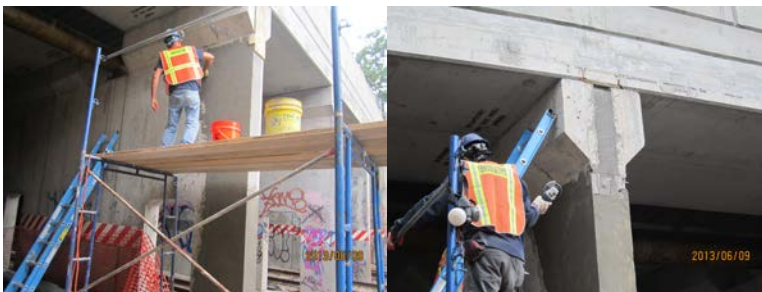
Smoothing the Upper Repaired Wall After Stripping Forms. Grinding the Repaired Wall.
