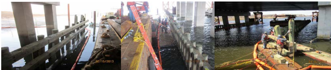
Fresh Creek Bridge in February, March, and April 2013: Timber Pier Protection Fender Under Construction, Turbidity Curtain, and New Pier.
