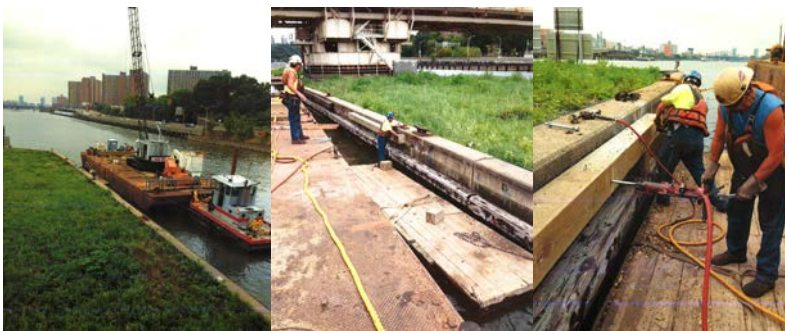
Macombs Dam Bridge over Harlem River: Fender System Repair.
