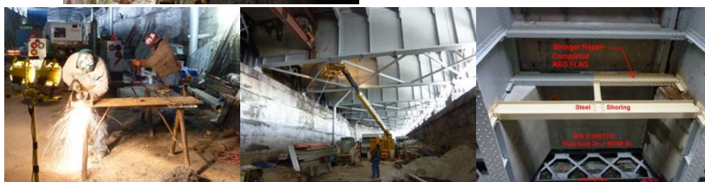
February 2011: Red Flag Stringer Repair at Riverside Drive Viaduct over West 158 th Street.
