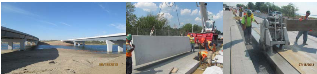
Paerdegat Basin Bridge in May 2013: New Bridges: Eastbound on Left, Westbound on Right. July 2013: Setting a Precast Concrete Median Barrier Section.
