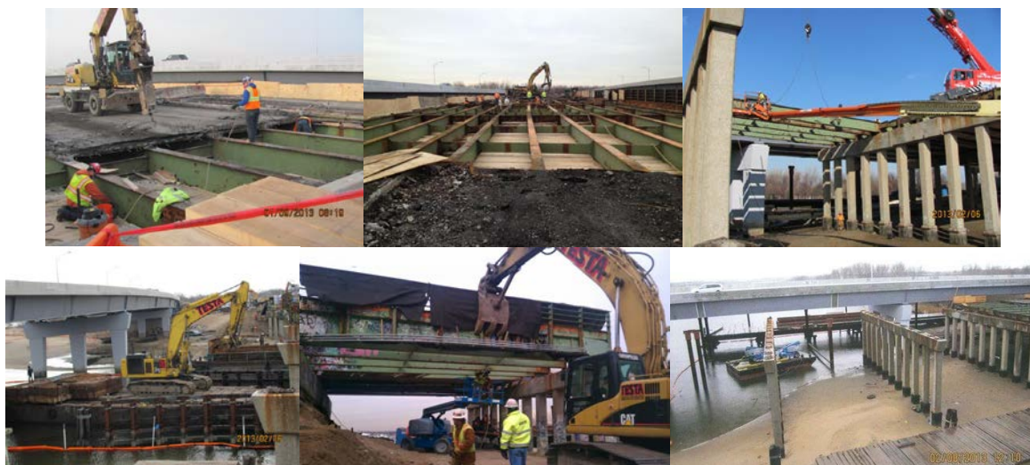
Paerdegat Basin Bridge in January 2013: Demolition of and Removal Bridge Deck at the Old Paerdegat Basin Bridge. The Timber Debris Shielding was Supported on the Lower Flanges of the Bridge Stringers. Demolition of Span 10 in February 2013.
