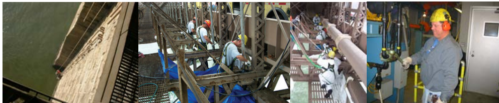
Repairing the Brooklyn Bridge Standpipe System, 130 Feet Below the Roadway. Maintenance Crew Conducting the Annual Cleaning and Lubrication of the Solid Rod Suspenders Spherical Bearings on the Brooklyn Bridge.
