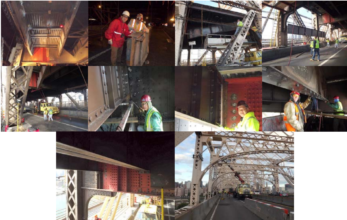
October 2013: Repairing the Ed Koch – Queensboro Bridge Stringers After a Truck Fire. Assistant Civil Engineer Andrew Hoang Inspecting the Measurements. Bridge Repairer and Riveters Charlie Zhao (Green Jacket), Yiu Liu (Yellow Jacket), Randall Palmenta, and Ignazio Trapani. Putting Up the New Beam. (Credit: Hany Soliman)
