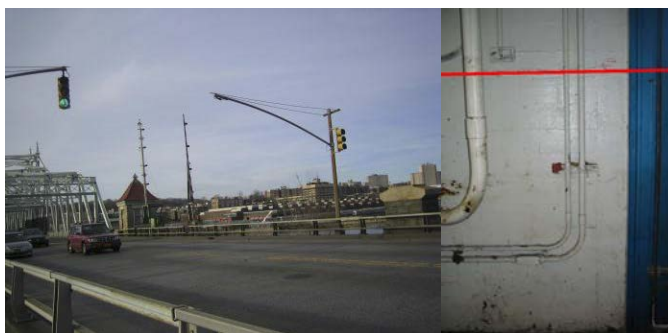
East End of the West 207 th Street Bridge - Missing Traffic Signal was Knocked Down by the Hurricane Winds. Borden Avenue Bridge Operator's House Basement Level - Depicted Flood Line was Approximately 5 Feet Above the Floor.
