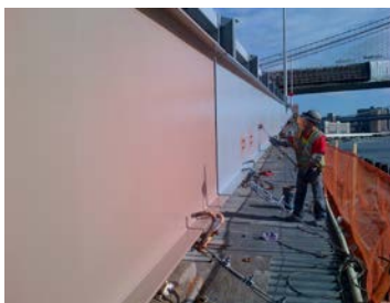
November 2013: Painting Fascia Steel on Ramp C.
