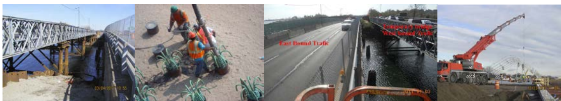
Fresh Creek Bridge March 2011: Westbound Temporary Bridge at Left, Existing Bridge at Right. July 2011: Concrete Pouring in Piles. November 2011: The Remaining Bridge Carrying East Bound Traffic and Temporary Bridge Carrying West Bound Traffic. (Credit: NYSDOT) December 2011: Commenced Installation of Winter Tent Enclosure for Stage IIB Concrete Bridge Deck Placement. (Tent Credit: Daniel Hom)
