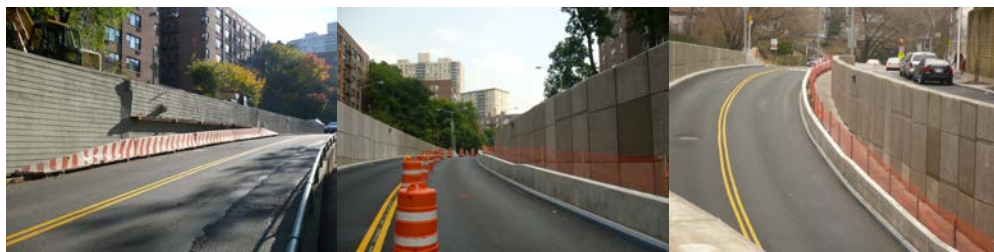
Kappock Street Retaining Wall in Riverdale, Before and After Repairs. The Existing 300-Foot Long Parallel Concrete Roadway Retaining Walls on Both Sides of Kappock Street Were Deteriorated and Leaning, and Were Replaced with New Modular Retaining Walls in the Summer of 2009.
