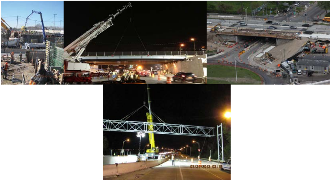
March 2013: Pumping Concrete for the West Abutment Wall. April 2013: Ironworkers Installing Structural Steel. East Abutment at Right. May 2013: Site Overview. July 2013: Nighttime Sign Structure Erection.
