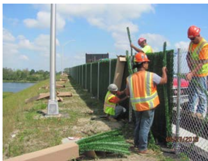
Installing the Privacy Glare Fence.
