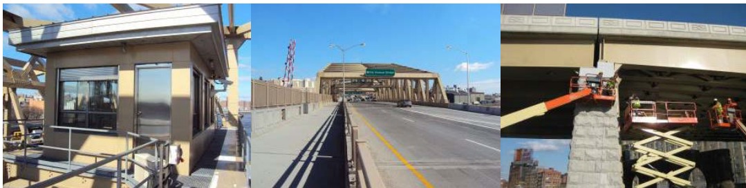
February 2013: Bridge Operator House. General View Taken From the West Side – Looking East. Pier 11- Continued installation of granite stone retrofit anchors.
