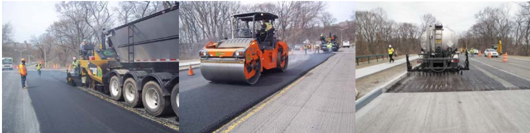
April 2013: Final Paving Operations - East and West Approach Roadways. Placing And Rolling Asphalt. Tack Coat.
