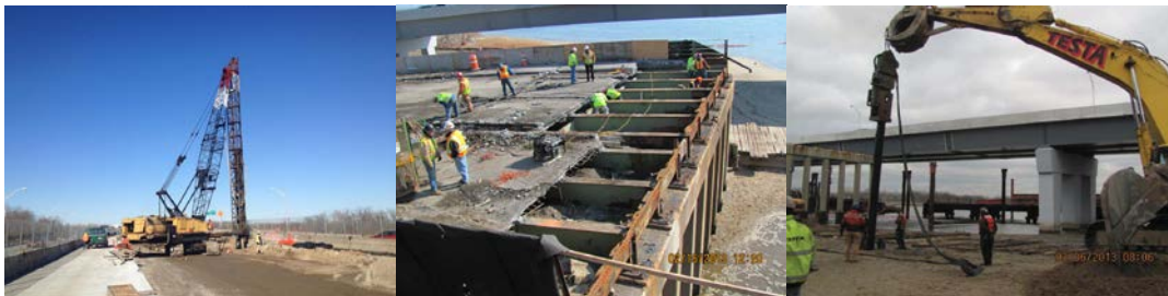
Paerdegat Basin Bridge in January 2013: Driving Support Piles for the Drainage System at the West Side. February 2013: Demolishing the Old Bridge. March 2013: Removing Temporary Piles for the Falsework Structure.
