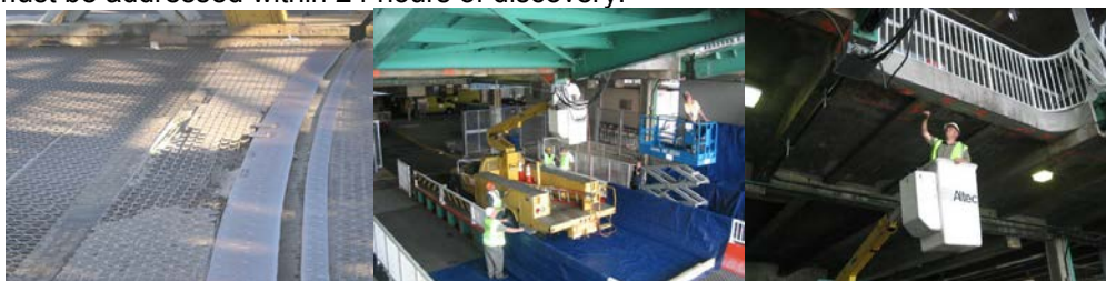
Example of PIA Safety Flag: Broken Grating. Executive Director of Bridge Preventive Maintenance and Repair Tom Whitehouse (White Hardhat) Ensuring the Proper Setup of Containment Procedures at the St. George Ferry Terminal Landing Slips Before the Masons Address A PIA Flag (Falling Concrete). Inspecting the Flagged Condition.
