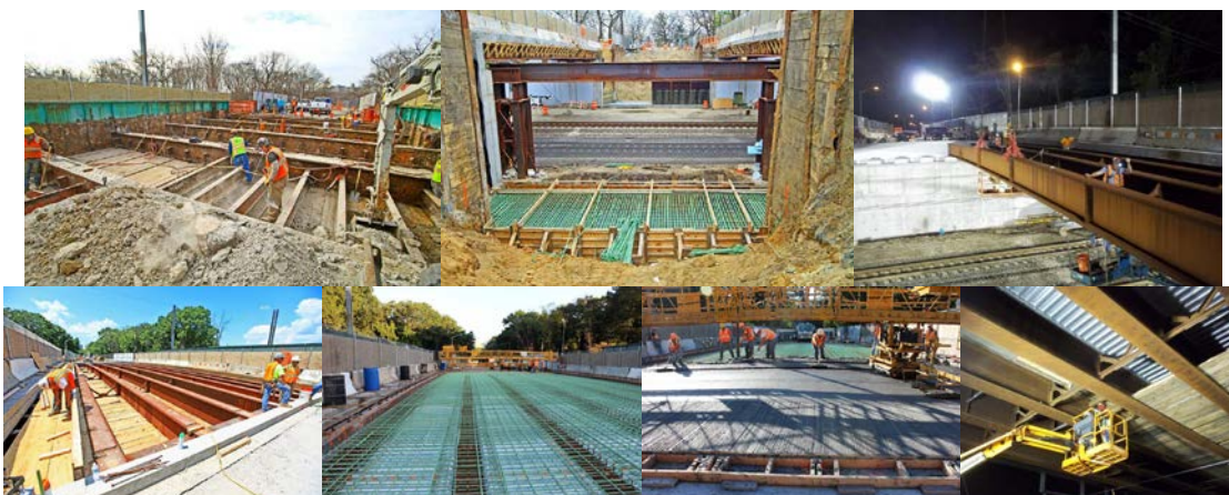
February 2012: Demolition of Existing Stage-2 Superstructure. April 2012: Existing Stage-2 Section of Bridge Demolished and Rebar for New Stage-2 Abutment Footing Placed. July 2012: Stage-2 Steel Erection. Formwork, Rebar Placement, and Concrete Placement for Stage-2 Superstructure Slab. December 2012: Removing Shielding and Formwork.
