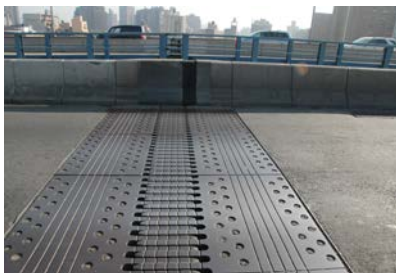
Manhattan Bridge Finger Dam. (Credit: Jagtar Khinda)
