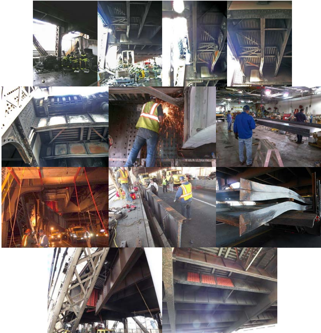
August 2013: Firefighters Examining the Damage. Repairing the Bridge Included Custom Designing the Steel Beams, as Well as Fabrication and Installation. Division Ironworkers Fabricated Two 26-Foot-Long, 1.5-Ton Beams in Their Brooklyn Shop. October 2013: Removing the Warped Beams. The New Beams.
