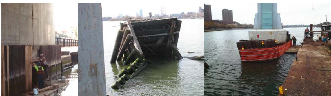
145 th Street Bridge Over Harlem River: Repairing the Horizontal Fender System. Wards Island Pedestrian Bridge: Collapsed Pier #6 Fender. Installing Protective Fencing.
