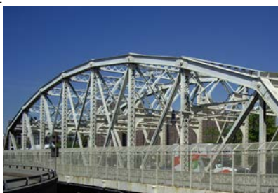
Macombs Dam Camelback Truss.
