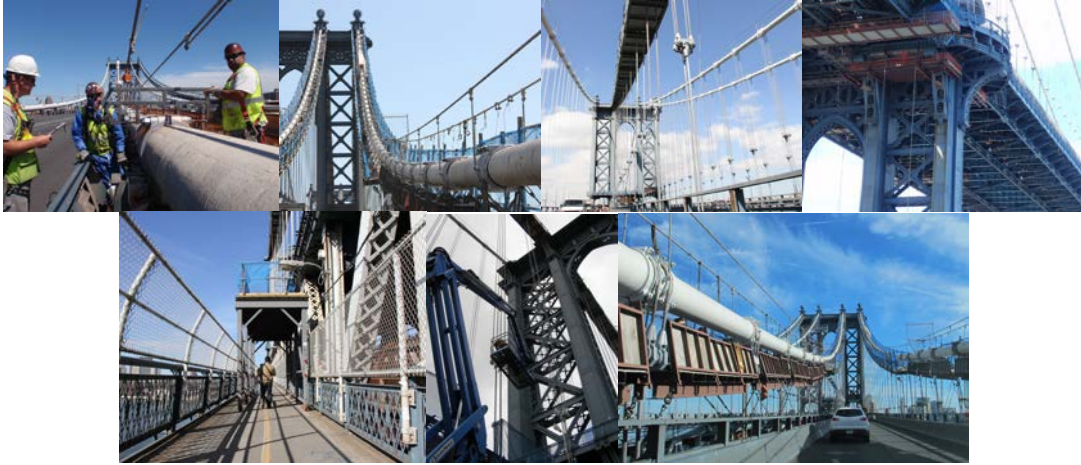
June 2012: Measuring New Cable Band Bolts. September 2012: Main Cable Work Platforms. New Suspenders Along Truss B. September 2012: Jacking Struts and Work Platforms. November 2012: Sidewalk Protection Sheds. April and September 2012: Manhattan Bridge Suspender Replacement. (Credit: Bojidar Yanev)
