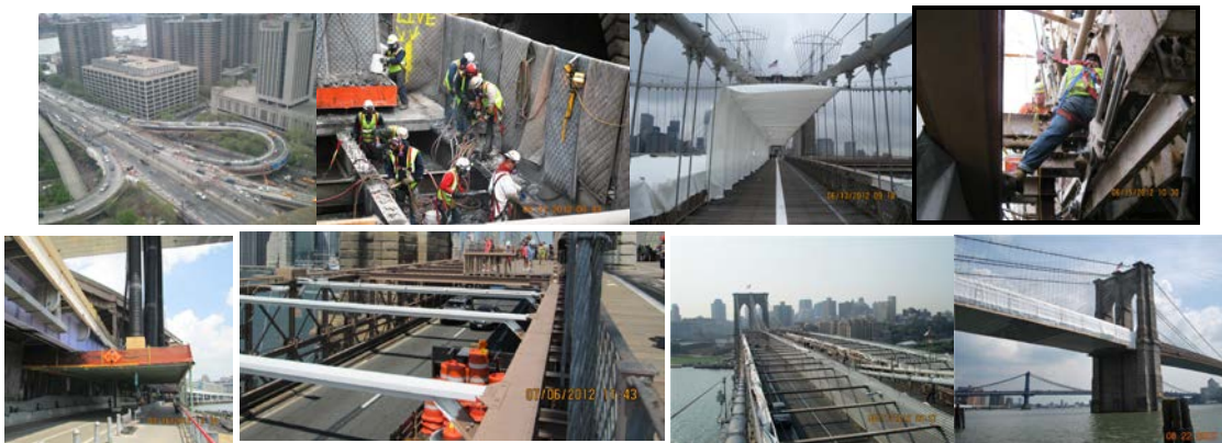
April 2012: Overview. (Credit: Maria Mikolajczyk) Manhattan Approach Existing Deck Demolition. June 2012: Brooklyn Side Span Netting Protection for Main Cable and Suspender Rope Painting. June 2012: Structural Steel Repairs. June 2012: Duct Hose Platform Over Esplanade. July 2012: Painting Brooklyn-Bound Top Struts. August 2012: Manhattan Main Span Vertical Wall. August 2012: Manhattan Side Span Containment at Manhattan Tower.
