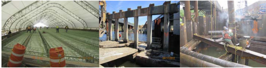
Fresh Creek Bridge in January 2012: Winter Tent Enclosure for Stage IIB Concrete Bridge Deck Placement. Fresh Creek Bridge in April 2012: Stage 3 Demolition of Piers of Old Fresh Creek Westbound Bridge. Workers Cutting off Excess Steel Pipe Casing for Cast-in-Place Concrete Piles at Future Westbound Bridge. Temporary Bridge at Left.
