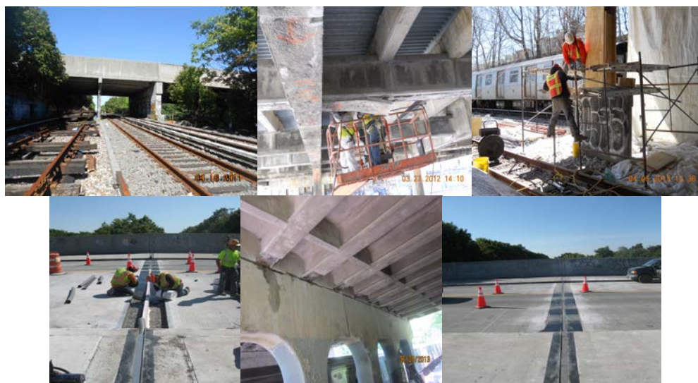
13 th Avenue Bridge. (Credit: NYSDOT) Repairing the Under Deck and Deck Joint. Bridge After Repair.
