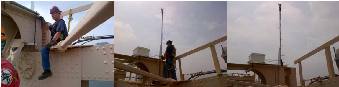
Bridge Repairer and Riveter Kevin Clarkson Installing Anemometers on the Ed Koch-Queensboro Bridge in July 2013. (Credit: Paul Schwartz)
