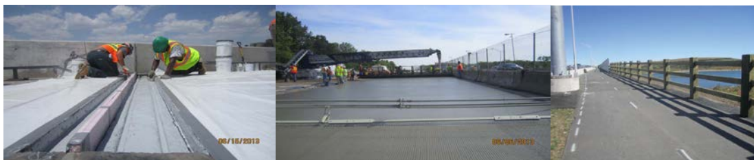
June 2013: Preparing Recess in the Deck Prior to Installation of Elastometric Expansion Joint. Placing Concrete for On-Grade Pavement at Bridge Approach by Means of Conveyor Belt. September 2013: Bicycle/Pedestrian Path on South Side of Bridge - Timber Rail on the Bridge Approach Leads to 7 Rail Bridge Rail on the Bridge.
