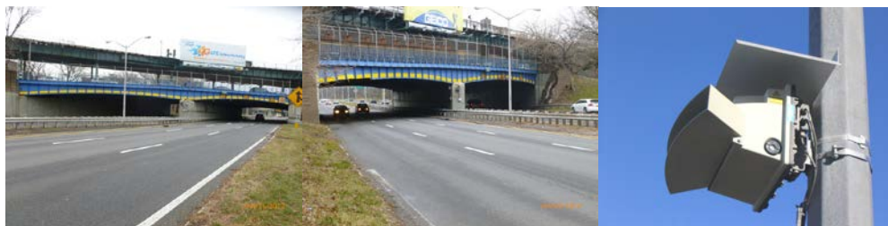
Westchester Avenue Bridge Elevation Left and Right in 2012. (Credit: NYSDOT) Overheight Sensor Unit on the Hutchinson River Parkway. (Credit: Roly Parroco)
