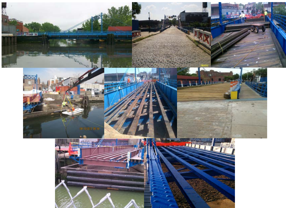
Carroll Street Bridge. (Credit: NYSDOT) Repairing the Deck, Approach, Fender, and Steel. Bridge After Repair.
