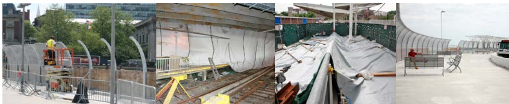
May 2013: Installing Pedestrian Fencing. June 2013: Containment For Steel Painting. Thin Deck Replacement. Ramp B Benches.
