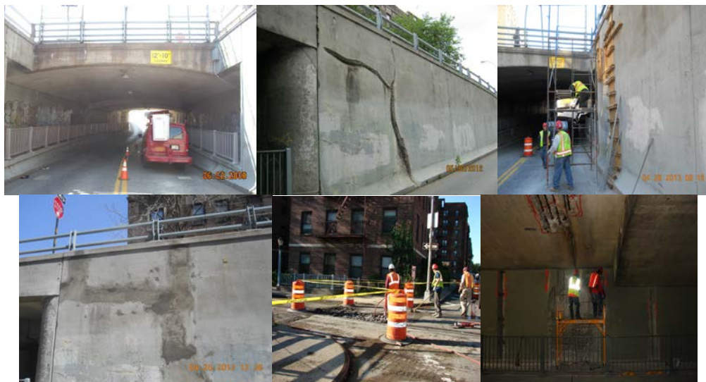
Jackie Robinson Parkway Bridge. (Credit: NYSDOT). Retaining Wall Repair – Before, During, and After. Deck and Joint Repairs. Under Deck Repairs.
