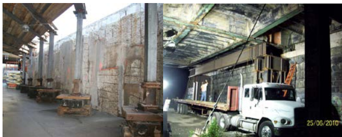
2010: Shoring of Stringers at Ramp D East Abutment (Staten Island Ferry Ramps) for Steel Repair Work. Installation of Shoring Towers at the Shore Road Circle Bridge.
