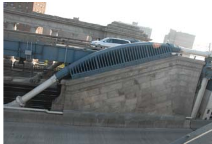
Manhattan Bridge Saddle. (Credit: Jagtar Khinda)
