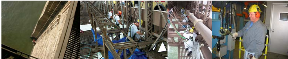
Repairing the Brooklyn Bridge Standpipe System, 130 Feet Below the Roadway. Maintenance Crew Conducting the Annual Cleaning and Lubrication of the Solid Rod Suspenders Spherical Bearings on the Brooklyn Bridge. 2 nd Photo - Oilers Steven Marxhausen, Rene Francis, Richard Morreale, Thomas McAuliffe, and Andrew Sorrentino. (Credit: Anatoly Orlov) Oiler T. McAuliffe at the 9 th Street Bridge
