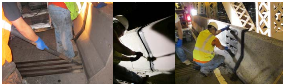
Expansion Joint Cleaning on the Williamsburg Bridge in September 2011. (Credit: Shaikh Islam)
