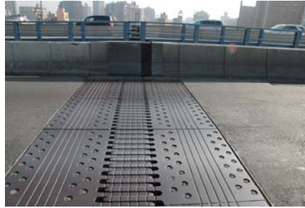
Manhattan Bridge Finger Dam. (Credit: Jagtar Khinda)
