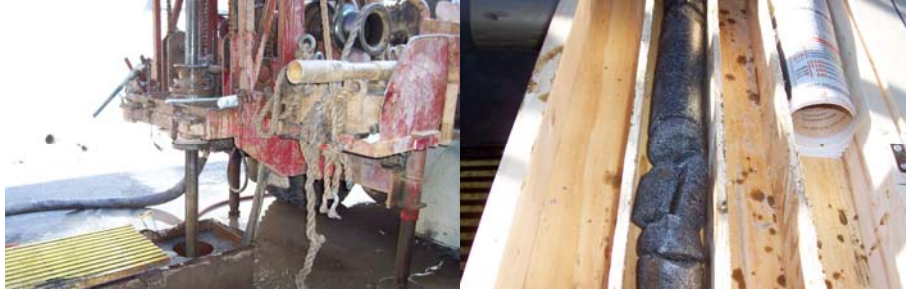
Conducting Soil Borings in 2008 as Part of the Seismic Retrofit Design of the Manhattan Bridge. Drilling to a Depth of Approximately 210 Feet to Obtain an 8-foot Long Hard Rock Sample. A 2 1/2 –Foot Long Hard Rock Sample Taken From a Depth of Between 202 and 204 ½ Feet.
