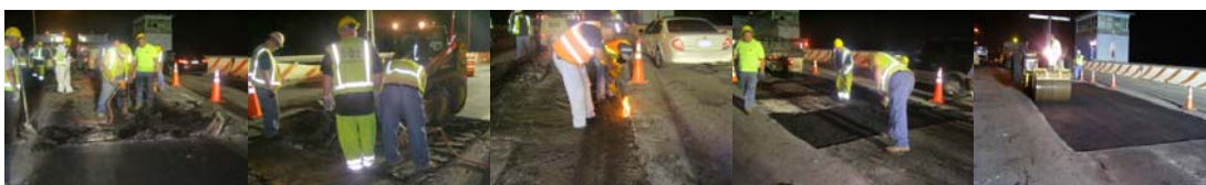
Resurfacing the Belt Parkway Bridge over Mill Basin on August 3, 2009. The Crew Completed a 13'x29' Cut in the Eastbound Center Lane, West Approach Spans. The Area Exhibited Rutting, Cracking and Excessive Patching. Breakout and Removal of Deteriorated Wearing Surface. Ironworker Assisting the Crew. Installation of New Asphalt. (Credit: Yousef Demis) Compacting the Asphalt With the Assistance of a Gasoline Roller Engineer From the Roadway Repair and Maintenance Division. (Credit: Ali Mozaffari)
