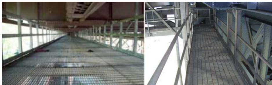
Ed Koch Queensboro Bridge Lower Level Flooring System Catwalk under Lower Level Queens Approach. Manhattan Bridge Brooklyn Tower Catwalk. (Credit: NYSDOT)
