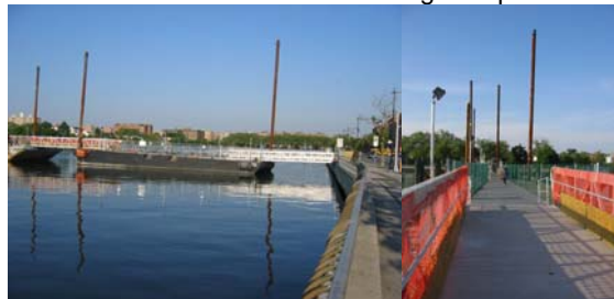
2005: Pontoon Bridge Used During the Emergency Reconstruction of the Ocean Avenue Pedestrian Bridge over Sheepshead Bay. (Credit: Russell Holcomb)
