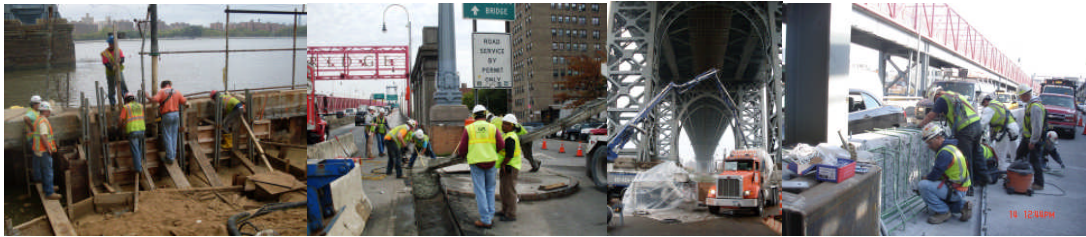
September 2011: Looking West at the Class GG Tremie Concrete Placement for the Kent Avenue Bulkhead Vertical Wall. October 2011: Looking East at the Placement of Concrete Footing for the New Lane 8 Precast Barrier at the Manhattan Plaza. October 2011: Looking West at the Concrete Placement for the Kent Avenue Yard Bulkhead Rehabilitation. November 2011: Looking East at the Rebar Installation for the Cast-in-Place Transition Barrier on the Brooklyn Approach.
