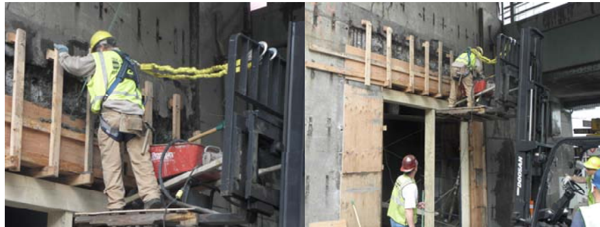
Performing Structural Repairs of the Entrance to the Cellular Structure at Joralemon Street Under the Brooklyn-Queens Expressway Triple Cantilever in June 2011. Loose Concrete was Removed and Replaced, and Rebar was Cleaned and/or Replaced. Cement Mason Victor Porowski Placing Concrete in the Forms While Standing on a Wooden Platform Raised by a Hi-Lo. He is Wearing the Appropriate Fall Protection Gear. Bridge Repairer and Riveter Brook Budd, Cement Mason Victor Porowski on Raised Platform and Lawrence Marks Operating the Hi Lo, and Carpenter Stephen Buckley. (Credit: Thomas Whitehouse)
