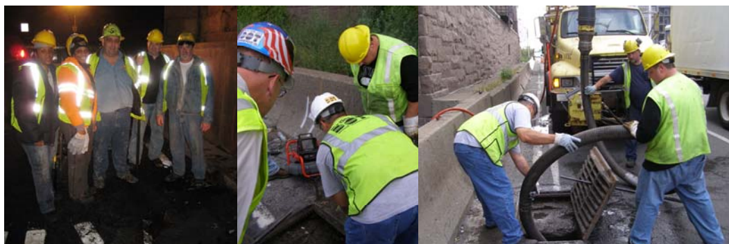
Drain Crew After Hand-Tool Cleaning the Clogged Catch Basins at Night on the Eastbound Brooklyn-Queens Expressway in April 2011: Highway Repairers Linda Rose and Sharon Britt, Supervisor Highway Repairer Joseph Turchiano, and Highway Repairers John Latona and Alfred Black. (Credit: Russell Holcomb) The "SnakeCam" is a Camera that is Fed Into a Drain/Sewer to Show the Crew What is Occurring. Executive Director of Bridge Preventive Maintenance and Repair Thomas Whitehouse, Supervisor Highway Repairer Anthony Irizarry, and Assistant City Highway Repairer John Tammaro Using the Camera on a Drain on the Eastbound Brooklyn-Queens Expressway in September 2011. Supervisor Highway Repairer Anthony Irizarry, Highway Repairer Michael Cunningham, and Assistant City Highway Repairer John Tammaro Using the Scupper Truck to Clean the Drain. (Credit: Paul Schwartz)
