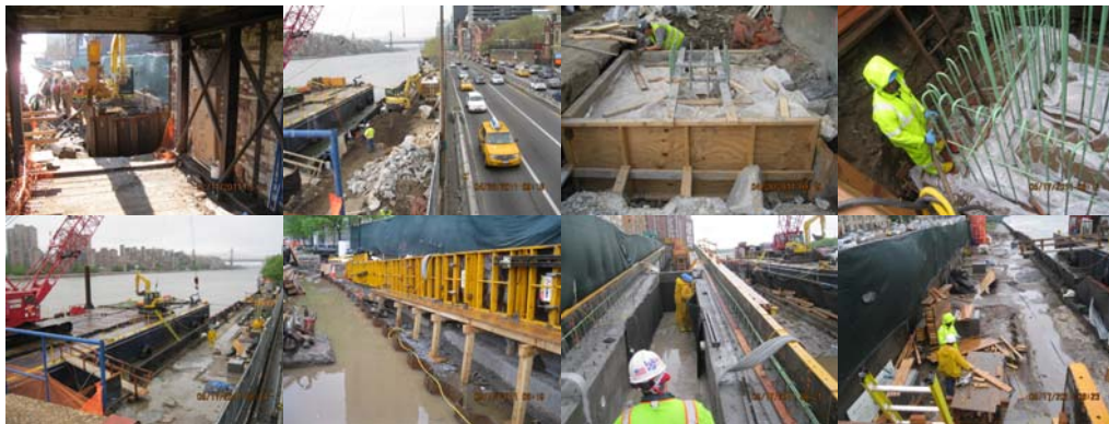
February 2011: Excavation Completed on East Abutment. The New Longer ADA-Compliant Ramp is Snug Against the FDR Drive. This Layout Improves Through Traffic Along the Esplanade. April 2011: Remove Bracing Abutment Piers and Pedestals. Continuing Excavation. May 2011.
