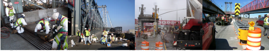
February 2011: Looking North at the Replacement of Existing Modular Joint Seals on the South Inner Roadway. April 2011: Looking North at the Replacement of Existing Modular Joint Seals on the North Outer Roadway. May 2011: Looking North at the Placement of a Temporary Barrier at the Manhattan Plaza in Preparation for the Clinton Street Traffic Signal Relocation Work. September 2011: Looking West at the Installation of the Brooklyn Approach Precast Median Barrier and Attenuator.
