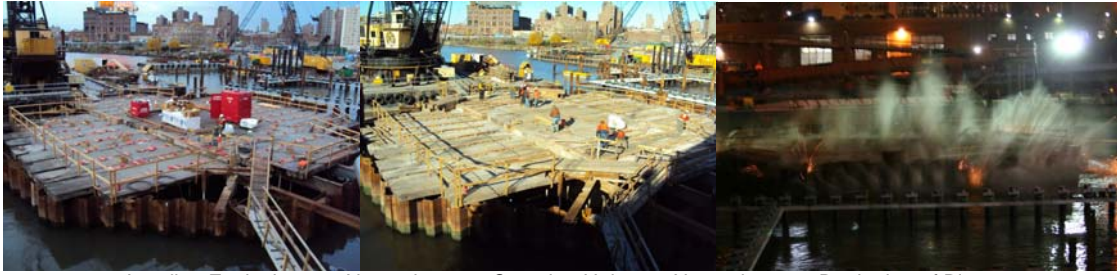
Loading Explosives on November 17. Covering Holes on November 18. Beginning of Blast.
