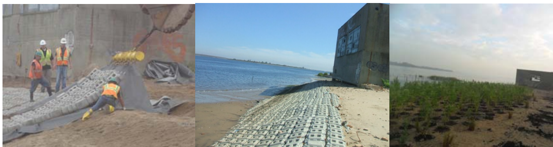
Summer and Fall 2011: Installing the Revetment. An Articulating Concrete Block Revetment System is Used as Slope Protection in Front of the Existing One Story Warehouse Building. Planting Bayberry; Groudsell Trees; Beach Plum Plants, and SwitchGrass.
