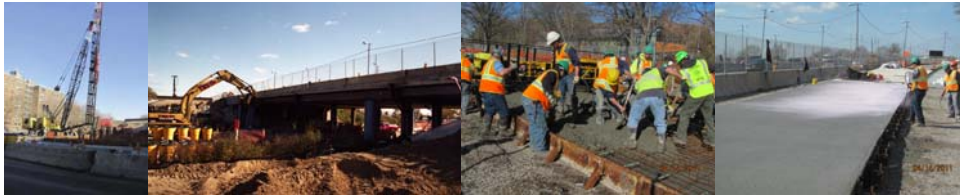
Rockaway Parkway Bridge in February 2011: Driving Steel Pile for Cast in Place Concrete Piles at East Abutment. March and April 2011.
