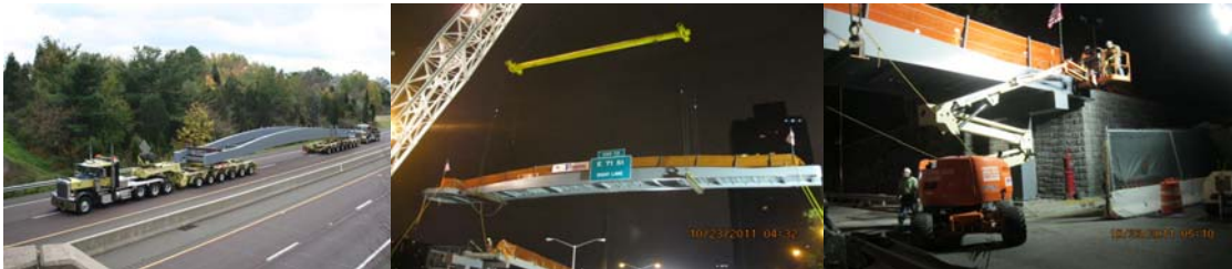
The New Bridge Span in Transit from Just North of Philadelphia to Jersey City. It was Then Loaded on the Barge and Brought up the East River to the Site. The Span Size was 26' x 135' and Weighed Approximately 80 Tons. New Main Span Steel Erection in October 2011.
