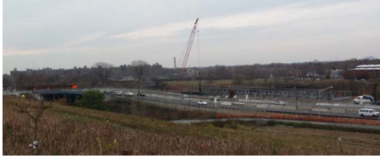
Fresh Creek Bridge in November 2010: Overview of the Existing Bridge and the Installation of the Temporary Bridge and Approaches North of the Existing Roadway. (Credit: Eric Callender)
