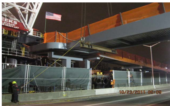
New Main Span Steel Erection in October 2011.
