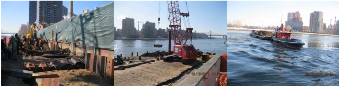
February 2011 at the East Ramp Area: Installing Interim Steel Sheet Piling on East Side, at Pier Footings # 10 and 11. Debris Loaded out Onto Barge and Removed by Tugboat.
