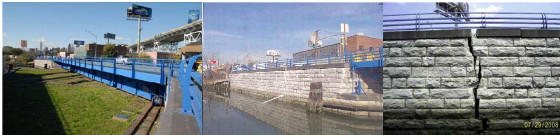
Borden Avenue Bridge. (Credit: Peter Basich) General and Close Up View of the Crack in the Wingwall. (2 nd View Credit: NYSDOT)
