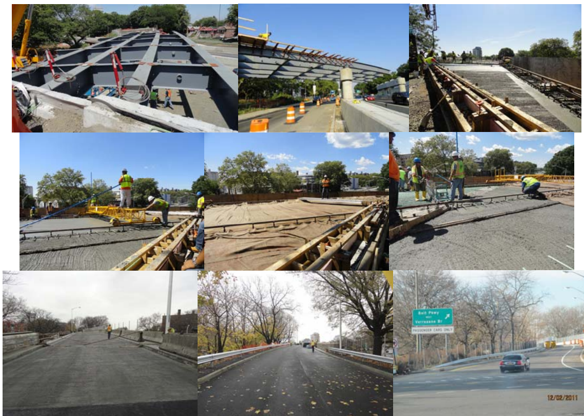
East 8 th Street Ramp in June 2011: Steel Installation for Span 1. July 2011: Installation of Steel Girders over the South Service Road and Eastbound Belt Parkway. August 2011: Concrete Deck Placement. November 2011: Completed North and South Approach Roadways. December 2, 2011: Bridge Open to Traffic.
