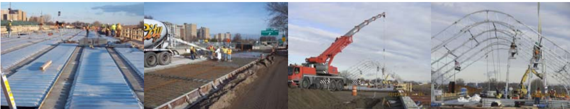
December 2011: Preparing the Decking for the Concrete Pour. Concrete Pours for Southeast and Northeast Roadways. Commenced Installation of Winter Tent Enclosure for Stage IIB Concrete Bridge Deck Placement. (Tent Credits: Daniel Horn)
