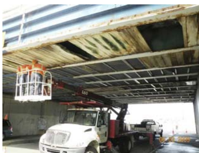
2009 Inspection: The Entire Underside of the Bay Ridge Avenue Bridge Deck is Shielded With Timber Planking and Steel Wire Mesh Netting. The Shielding was Temporary Removed to Perform the Inspection of the Deck. Shielding was Replaced After the Inspection. (Credit: NYSDOT)
