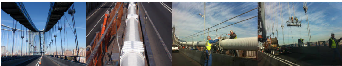
November 2011: New Suspender Assemblies Along 'C' and 'D' Trusses (Temporary Platforms Shown Above). Main Cable Wrapped With Walking Surface. Power Tool Cleaning Cable Circumferences and Grooves.
