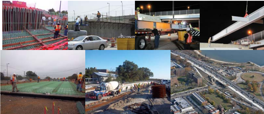
May 2011: Preparing Rebar for Northeast Abutment Footing. June 2011: New Footing and Wing Walls at Northeast Side. July 2011: Constructing East Abutment, North Side of Belt Parkway. Completing the Steel Erection for the Northern Section in August 2011. (Credit: Daniel Hom) September 2011: Installing Reinforcement Steel for Stage 2 Westbound Lane Decking. October 2011: Pouring Concrete for Northeast Approach. Aerial View in November 2011.
