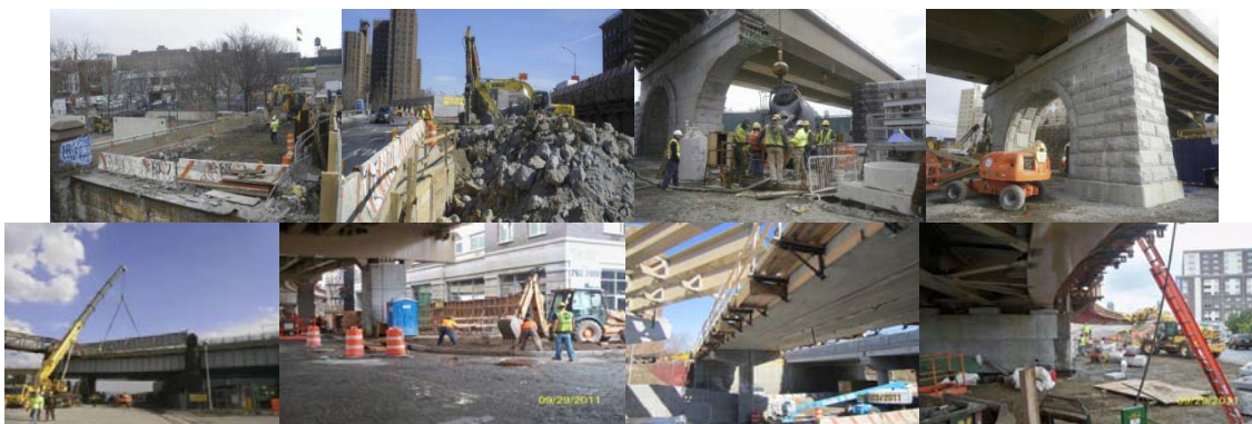
March 2011: Completed Excavation and Disposal of Existing Approach Slab and Roadway Pavements at B Ramp, Stage III. . Completed Excavation and Disposal of Existing Willis Avenue Abutment Footing and North Retaining Footing for Stage 5B Construction. Stage III Caisson Concrete Placement at Caisson #2 at Pier 11. Setting Granite Stone Facing at Pier 11. Finished Stage VB Removal of Steel Girder at South Bay at Existing Span 15. September 2011: Construction of Sidewalk at Bruckner Boulevard. February 2011: Pedestrian/Bicycle Bridge and Ramp to Major Deegan Expressway. September 2011: Granite Installation for Approach to Connector Ramp.
