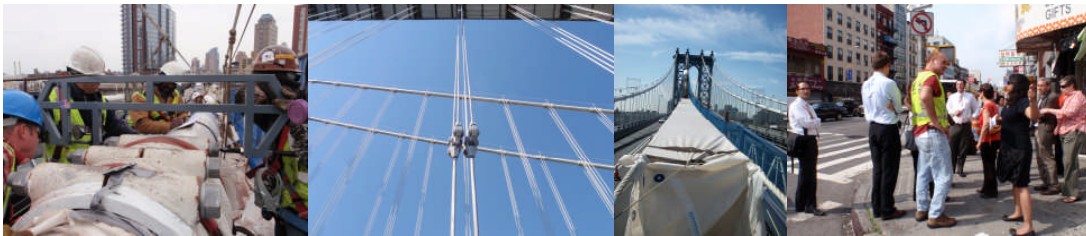
April 2011: Checking Bolt Tension in New Cable Band Bolts. New Suspender Assembly on 'C' Truss. May 2011: Painting Main Band Cables. June 2011: Reviewing the Bikeway Detour – Assistant Commissioner of Traffic Management Ryan Russo, Director of Bicycle and Pedestrian Programs Joshua Benson (Back Turned), Manhattan Bridge Engineer-in-Charge Brian Gill, Bicycle Program Coordinator Hayes Lord, First Deputy Commissioner Lori Ardito (Orange Top), Deputy Commissioner Gerard Soffian, and Chief Staff Manager/Executive Director of Community Affairs Joannene Kidder (at Right).
