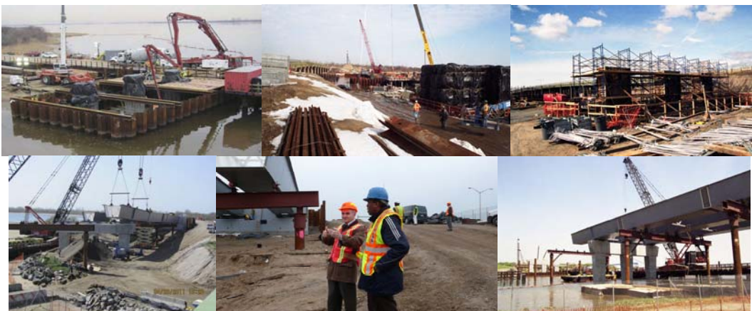
February 2011: Pumping Concrete at Paerdegat Basin Cofferdam for Pier No.3. February 2011. March 2011. April 2011: Setting Tub Girder Sections at Eastbound Bridge Between West Abutment and Pier No. 1. Civil Engineers Edvard Jeamgocian and Ferdinand John Observing the Operation. May 2011: Eastbound Bridge – New Concrete Pier No. 2 and Temporary Supports for Tub Girders.
