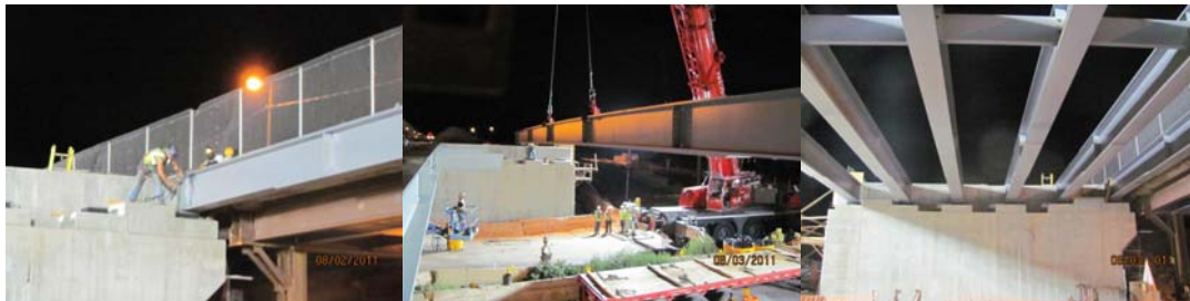
Completing the Steel Erection for the Northern Section in August 2011. (Credit: Daniel Hom)
