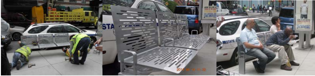
Bridge Repairer and Riveter Ignazio Trapani Drilling the Holes for the Concrete Anchor Bolts to Hold the Bench Securely in Place. Bridge Repairer and Riveters Ignazio Trapani, Fabian Del-Tongier and Salvatore Dimuro - Final Tightening of the Bolts and Installation of the Cover Plates to Hide the Connections. (Credit: Thomas Whitehouse) Bench Prototype and Testing by Citizens.
