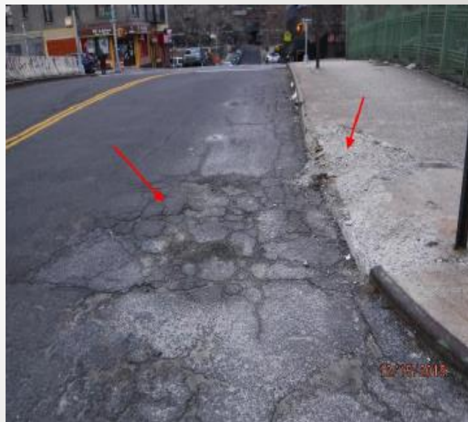
DETERIORATED PAVEMENT SPALLED SIDEWALKS
