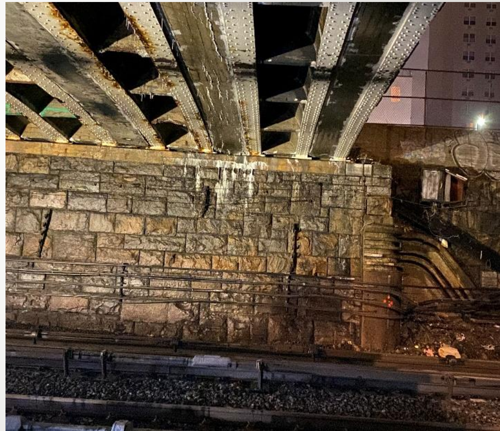
ABUTMENT STONE JOINTS IN POOR CONDITION
