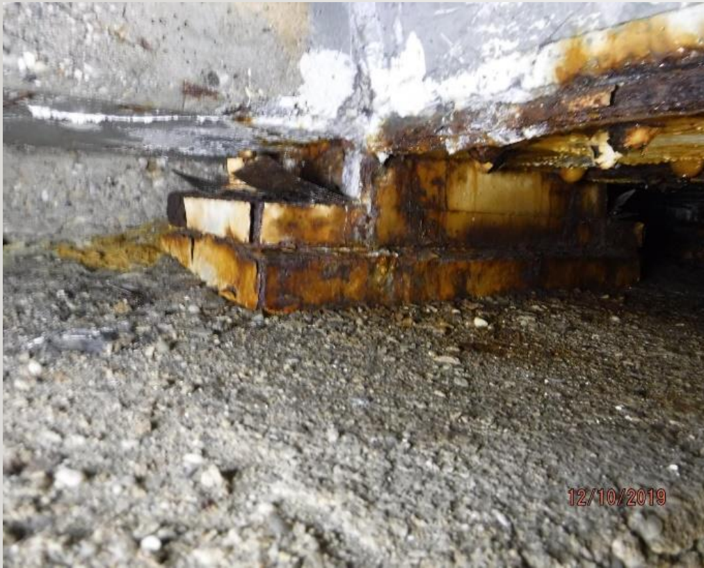
DETERIORATED BEARINGS
