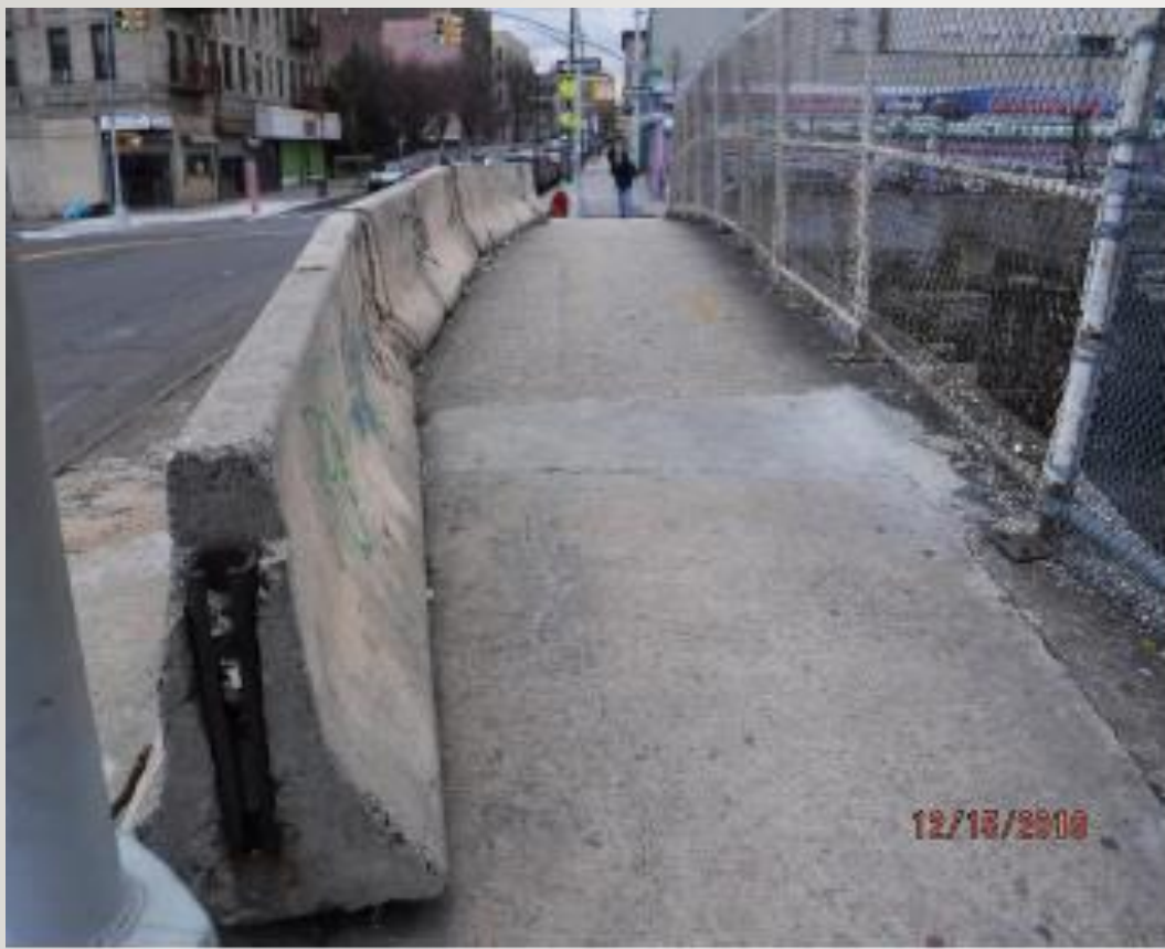
NO TRAFFIC RAILING AT SOUTH SIDEWALK
