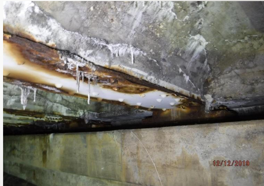
CORROSION AT GIRDER (VISIBLE BOTTOM FLANGE)
