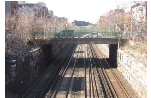
East 188 th St Bridge
