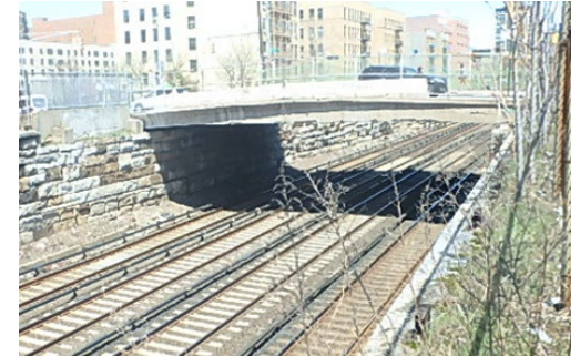
East 183 rd St Bridge
